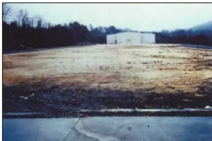
Oak Ridge Warehouses site after Phase 2 remediation, December 1992 (DOE Digital Archive).
