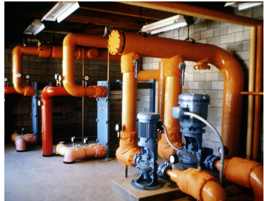
Heat exchangers and circulation pumps for the geothermal district heating system in Klamath Falls, OR. Photo by Geo-Heat Center (NREL Pix 03694)
