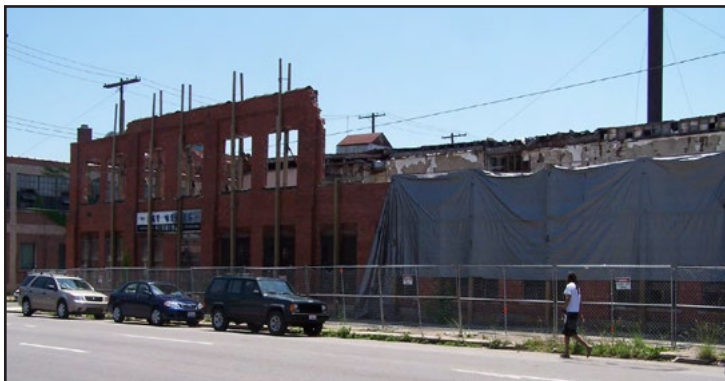
Main manufacturing building at the former B&T Metals site (2006).
