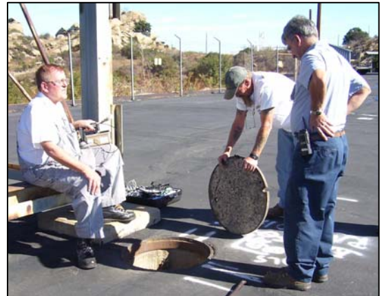
Photo 1. Manhole B-12 viewed from the southwest.
