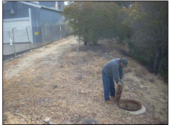
Photo 1. Manhole B-11 viewed from the north.
