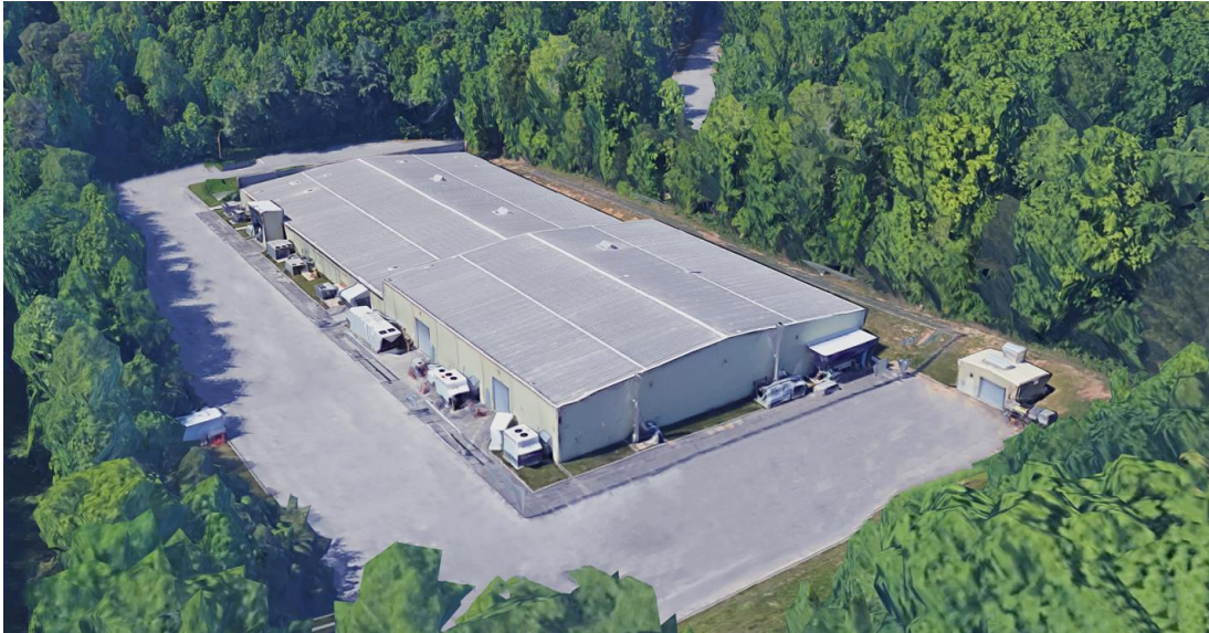
Figure 2-1. Test and Demonstration Facility (looking east)
