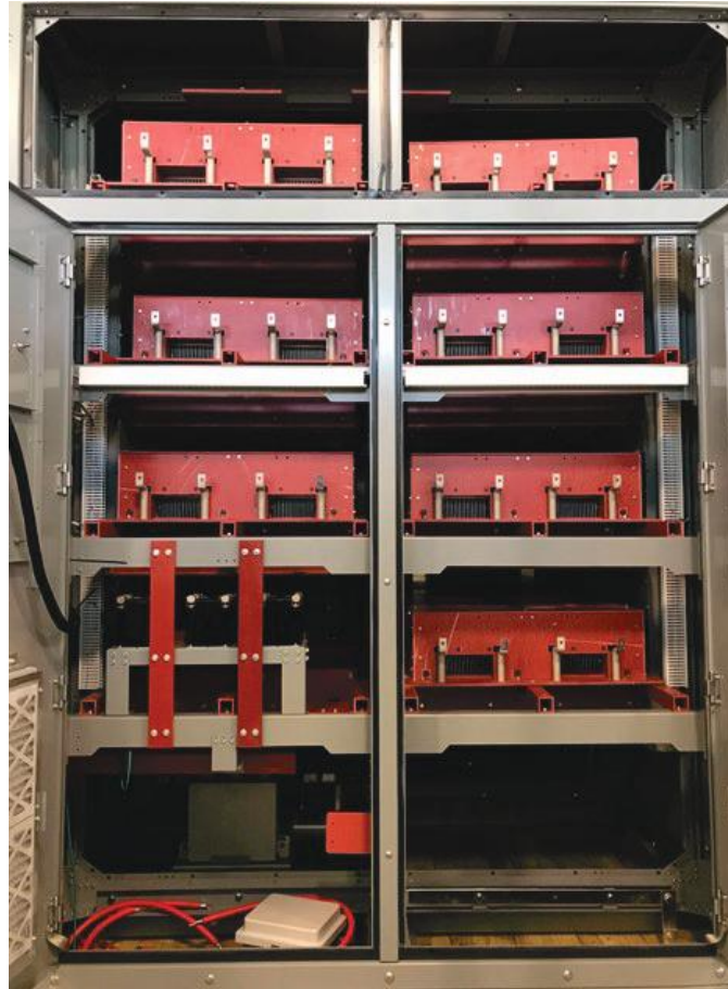
Figure II.1.8.6 DC – DC modules fitted inside the cabinet.
