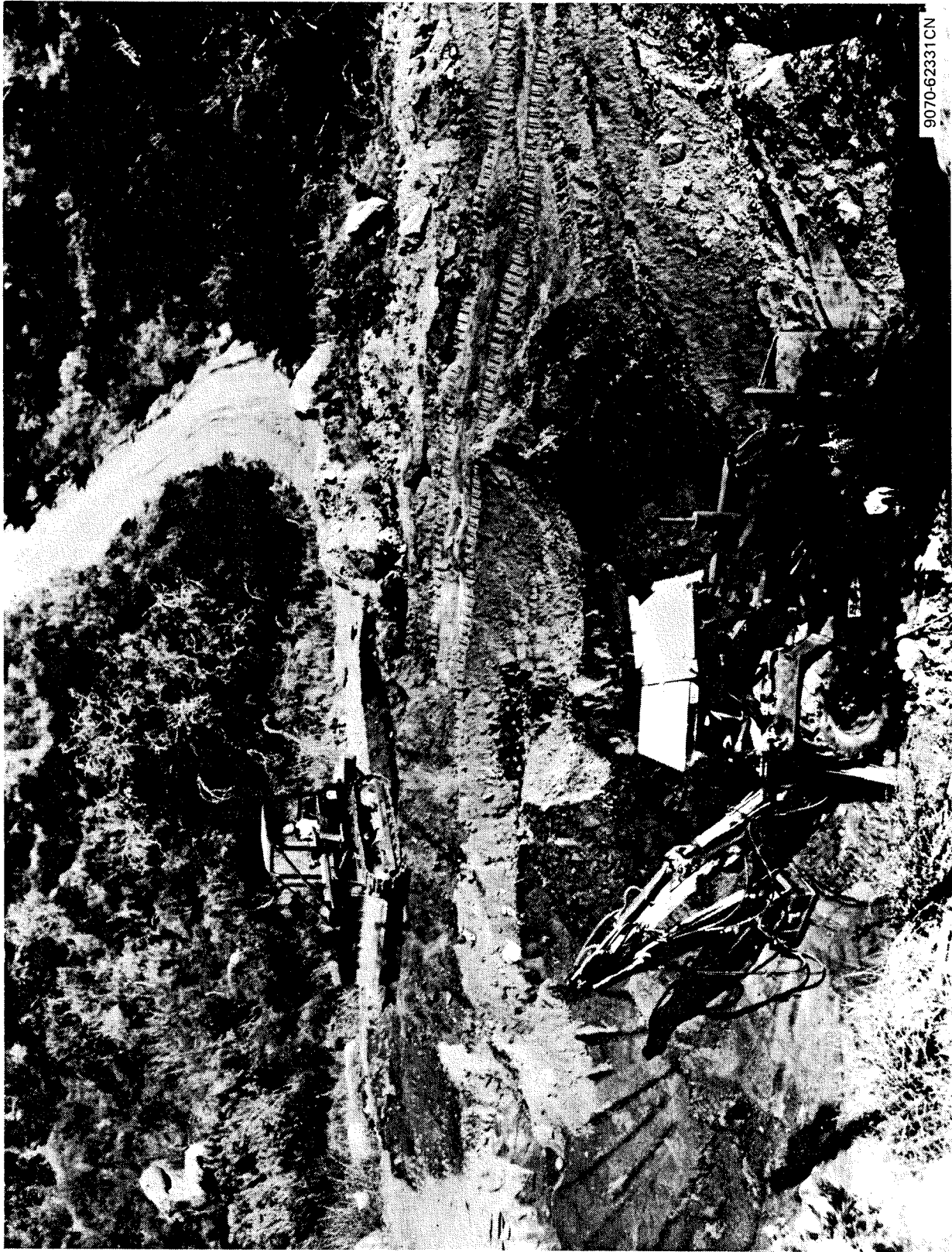
Figure 22. Compaction of Clean Overburden
