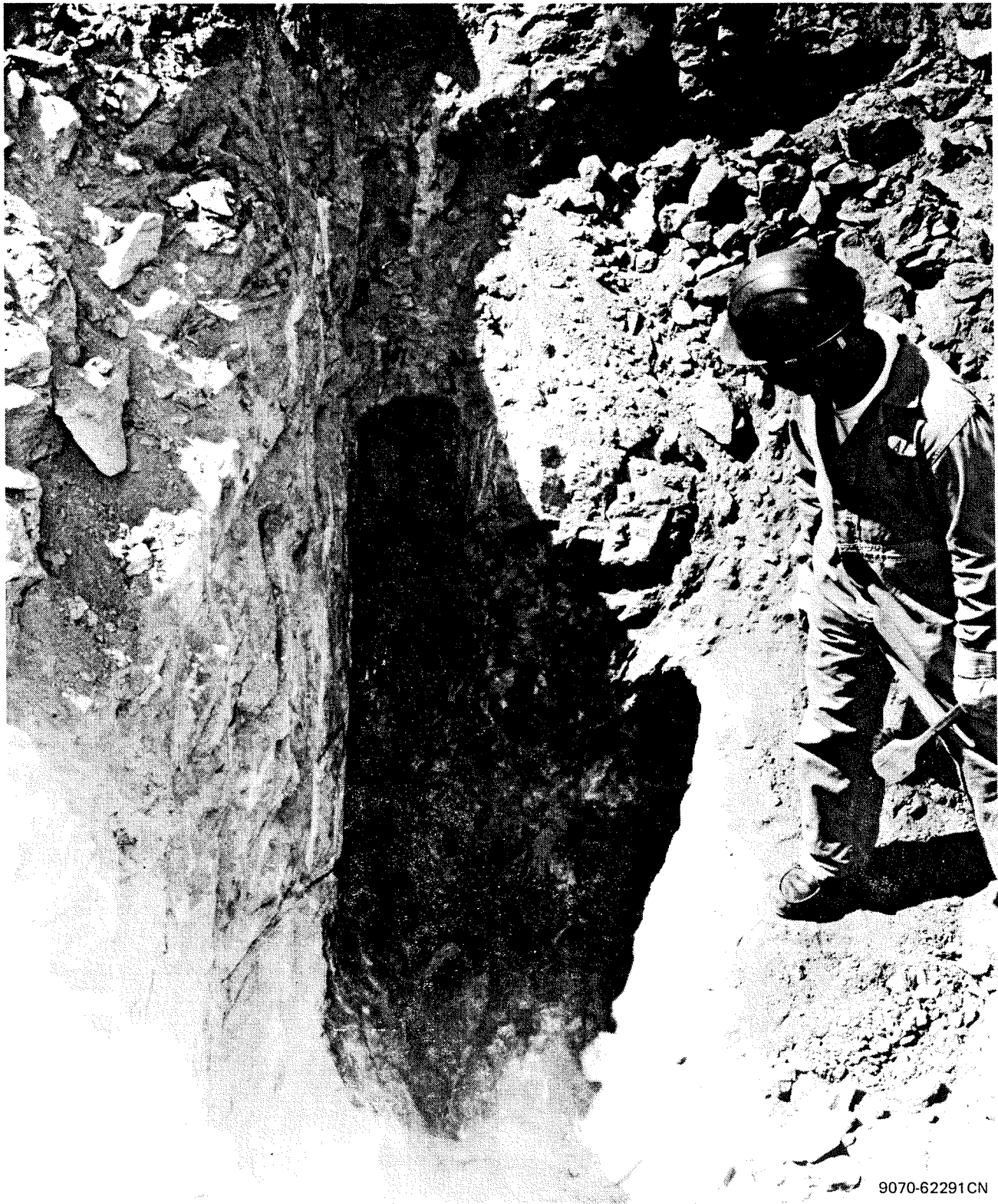
Figure 20. Close-up Photograph of Contamination Removal from Rock Fracture
