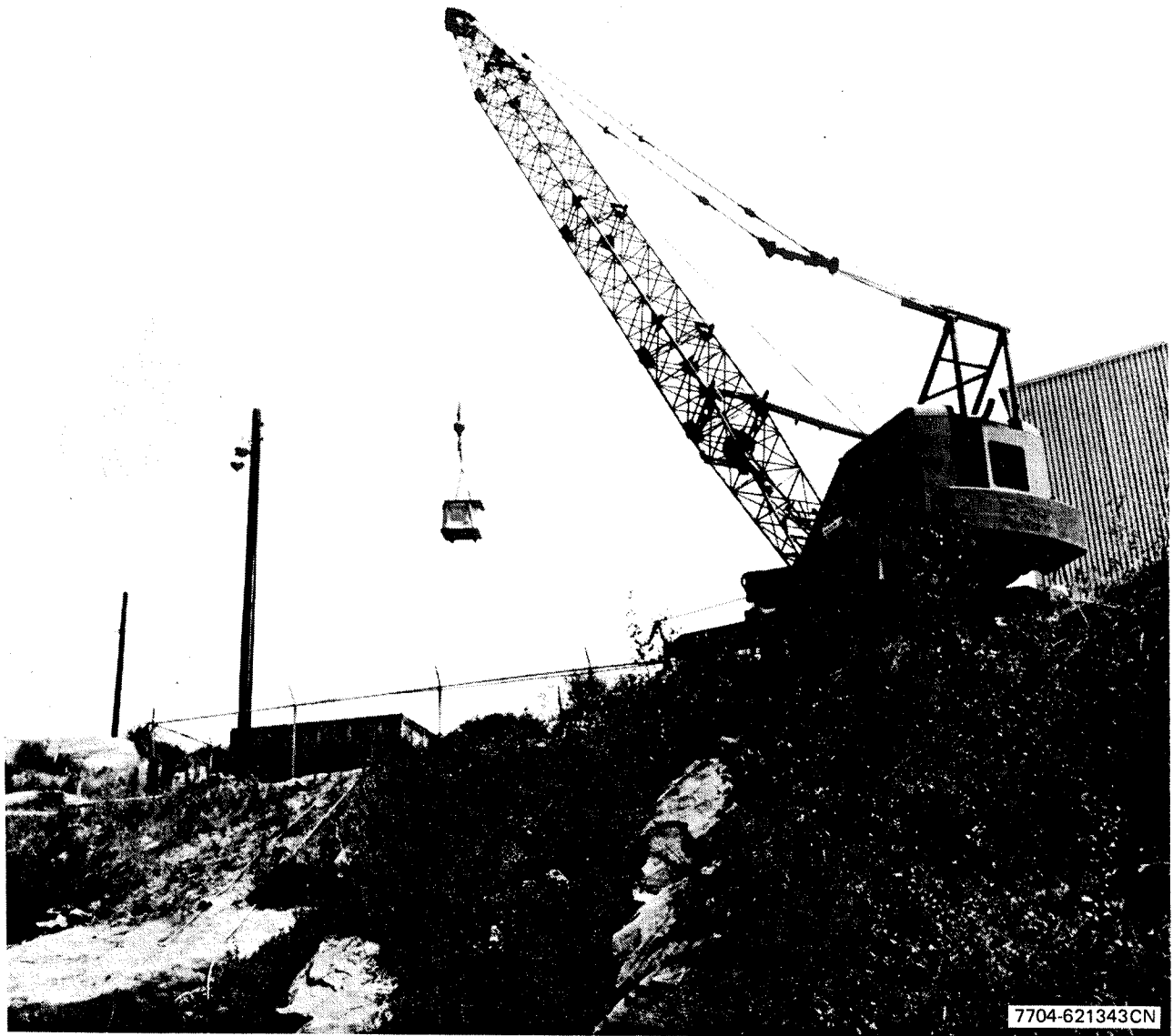
Figure 16. Crane Hoisting Soil Container from Leach Field
