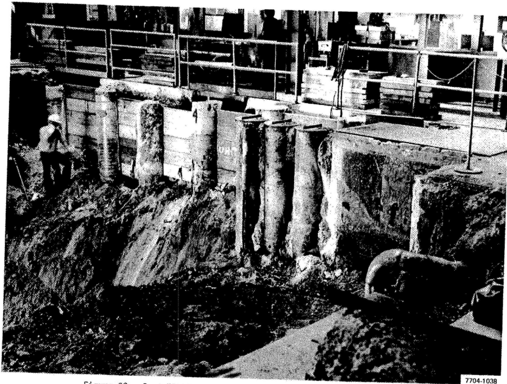
Figure 53. Installation of Wooden Shoring in High-Bay Retaining Wall
