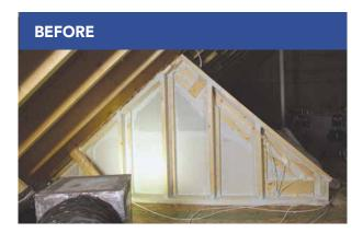
Install durable backing material into any large gaps before applying spray foam to prevent foam from leaking into conditioned space. All surfaces in contact with foam should be free of dust and debris. Ventilate the work space according to manufacturer specifications to ensure workers and occupants are protected from spray foam vapors during and after installation.
