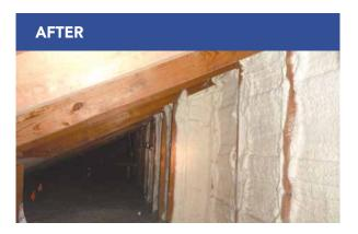
Spray walls as evenly as possible to the prescribed thickness to achieve the desired R-value. Consult with the manufacturer to determine the correct R-value per inch as it can vary by manufacturer.
