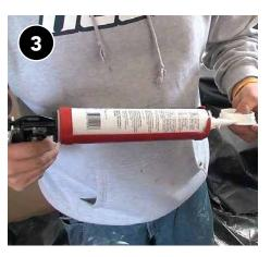
Apply a bead of caulk around the edge access hole plugs or seal holes using an alternative method that is aesthetically acceptable (e.g., foam plug covered with spackling compound).
