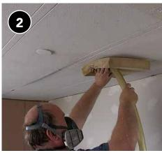
Blow loose fill fiberglass insulation to the correct density while ensuring complete coverage.
