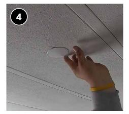
Close and seal all access holes to ensure an airtight and durable repair.
