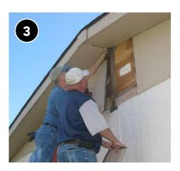
Remove or carefully fold the gable end cladding material to access the attic. Access can also be achieved by removing the existing gable vents or installing new ones.
