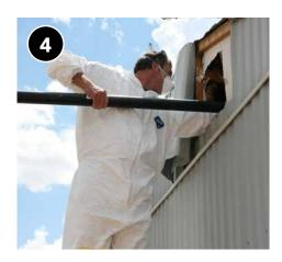
Insert the insulation fill tube as far as possible, moving the tube side to side while slowly retracting it to ensure adequate insulation coverage. If a marriage wall is present, use this technique on each side of the wall.
