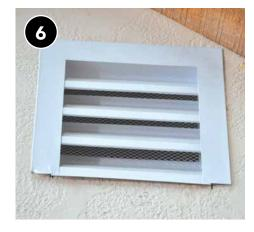
Depending on the method of access, reseal gable end cladding material or install vents with mesh screening no larger than 1/4 inch. Repeat all steps from the other end as needed to ensure adequate coverage.
