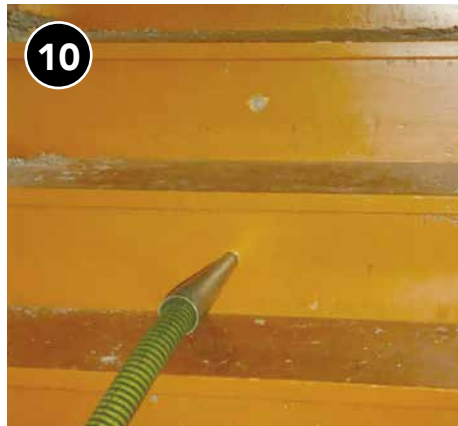
10 If backside of stairs already have backing material, blow insulation into cavity behind stairs.
