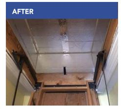
Attic pull-down stairs are safely and durably sealed and insulated to prevent air movement and reduce heat transfer.
