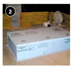
Insulate top and sides of dam cover, to appropriate R-value. Use materials that meet the requirements of the applicable fire safety code (e.g., thermal or ignition barriers).
