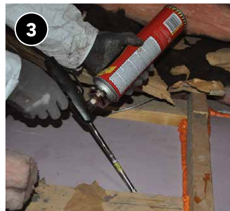
3 Ensure air sealing work is complete prior to adding insulation.
