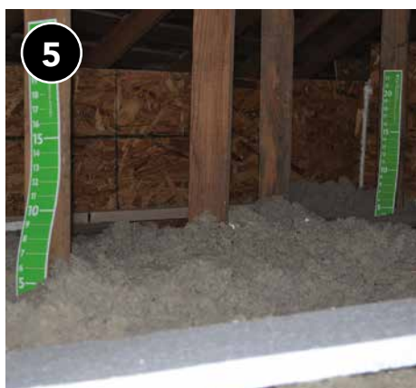
5 Insulation depth rulers installed, 1 per 300 square feet.
