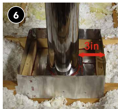
6 Dams are built around heat sources and air sealing is completed using approved materials (e.g., metal flashing, high-temperature rated sealants, etc.). The damming should be higher than the finished depth of any new insulation. Note that the clearance distance from damming to insulation can vary; follow guidance from the authority having jurisdiction.
