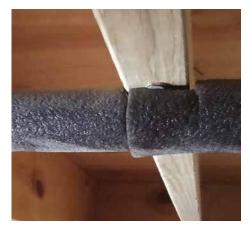
When path is partially obstructed or curved, shape insulation to the location to eliminate gaps.
