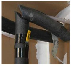
Insulation should be continuous with no gaps. Cut pieces at a 45 degree angle to join two pieces of a 90 degree angle.
