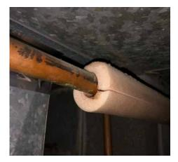
Insulate pipes to a minimum R-3 at least 6 feet from the water heater on both hot and cold lines. Use pipe wrap with an interior diameter sized correctly to fit the pipe.
