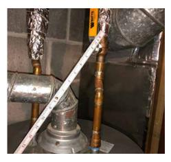
Keep insulation back at least 6 inches from draft diverter and single wall pipe.
