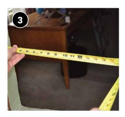
Measure rough opening for pane, size pane 1/8–3/16 inches smaller than the opening to ensure proper fit and minimize the potential of the glass cracking during installation.
