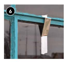
Temporarily hold new pane with tape and carefully install new push points.
