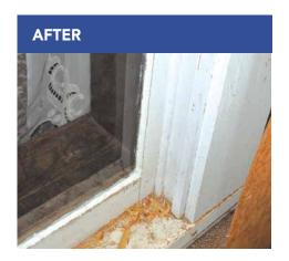
Newly installed glass is sealed to prevent air and water leakage.
