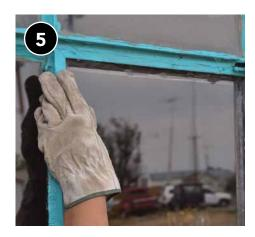
Install new glass, using tempered where code requires, that meets or exceeds the specifications of the previous glazing.
