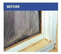
Broken, cracked, or missing glass breaks the pressure and thermal boundary.
