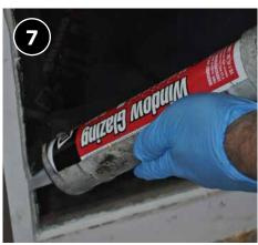
Install glazing compound or sealant at all edges of the glass.
