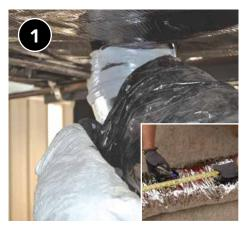
Pull excess insulation tight to cover and insulate the exposed boot or measure and cut a new piece of duct wrap insulation to fit.
