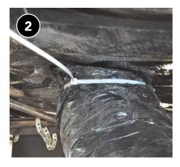
Secure the insulation in place, then seal around the boot to plenum connection with mastic to ensure a complete vapor retarder seal.
