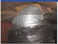
Exposed duct boots are a prime location for energy loss when ductwork is located in an unconditioned space.
