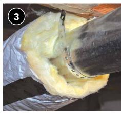
Ensure insulation is not compressed.
