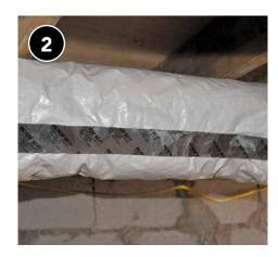
Tape joints to secure insulation in place.
