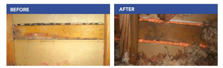
**SEAL TOP PLATES** Seal perimeter at all gaps and extend sealant up onto adjacent materials.
