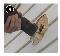
Locate exterior vent based on duct run and size hole less than 1/2 inch larger than duct.
