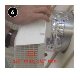
Chose appropriate exterior termination to match size of duct while minimizing water and pest intrusion. Seal around exterior termination as needed.
