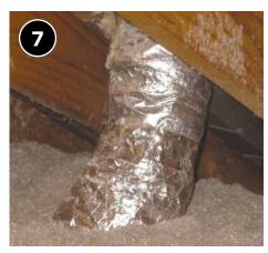
Insulate ducting that runs through unconditioned space to R-8.
