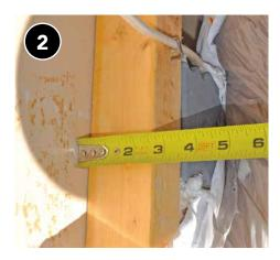
Measure the cavity depth, width, and length.
