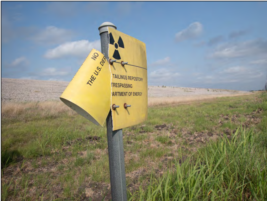
PL-2. Broken Perimeter Sign P62
