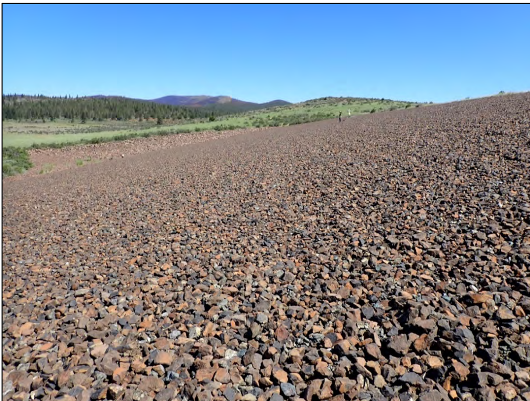
PL-8. West Side Slope of Disposal Cell
