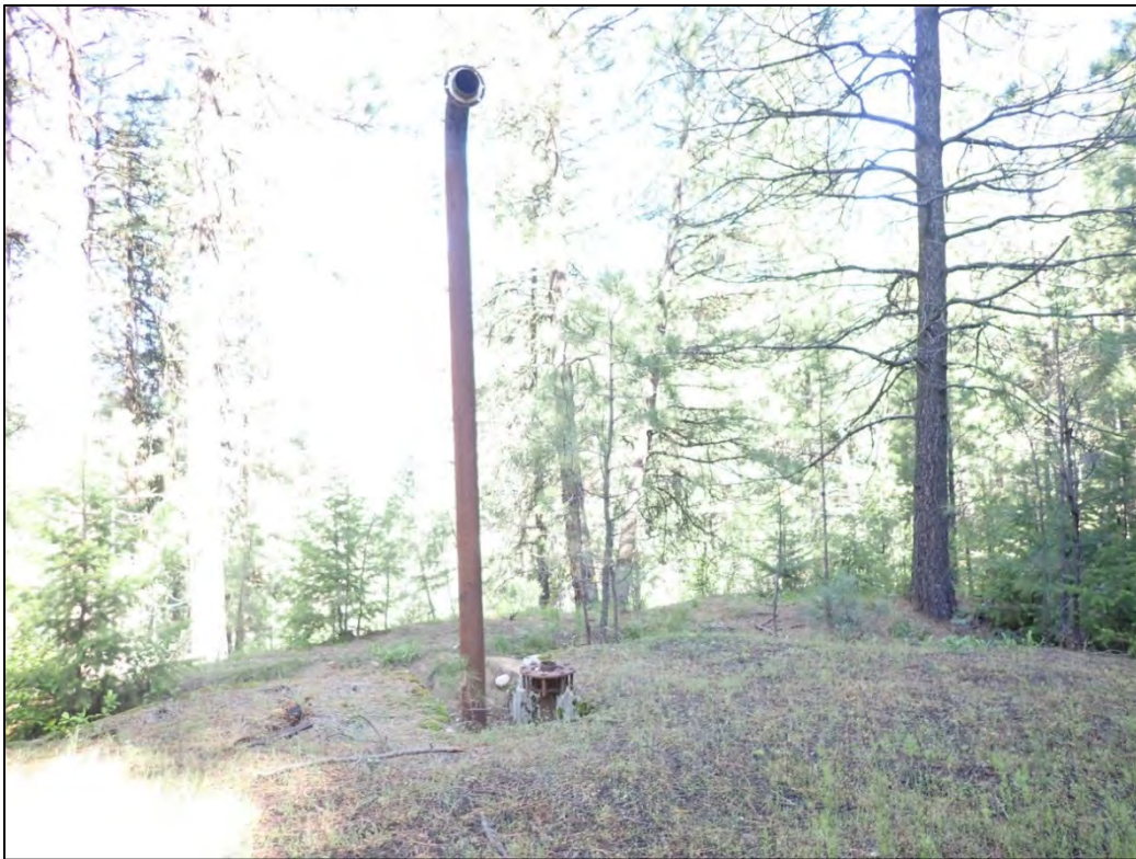
PL-8. Piping from Former Mill
