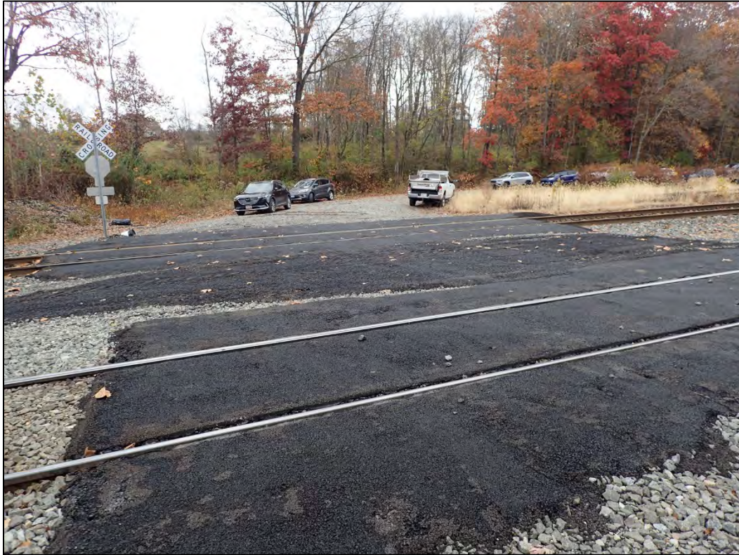
PL-1. New Blacktop Crossing to Site Entrance
