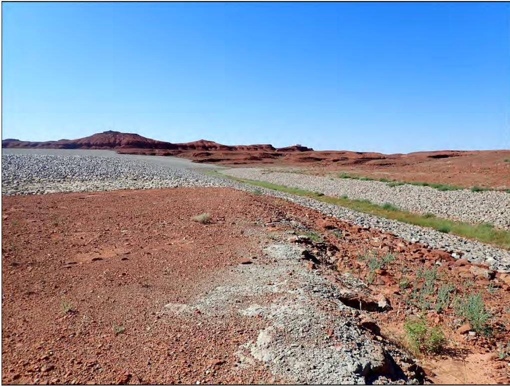
PL-9. Vegetation in the Northeast Toe Drain
