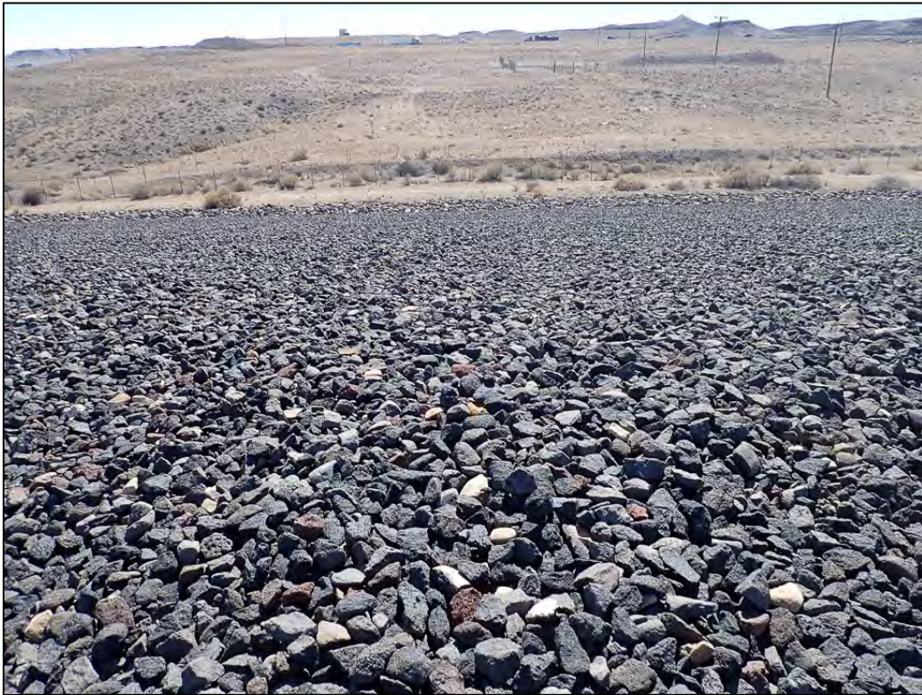
PL-9. Southeast Side Slope of Disposal Cell
