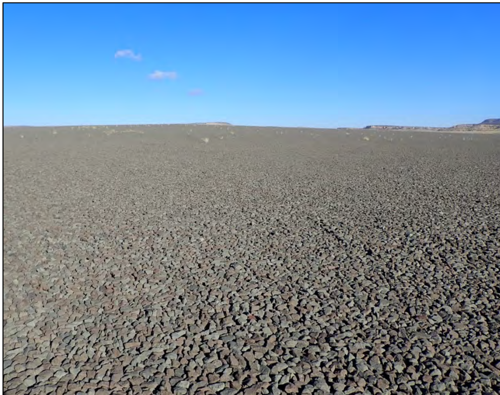
PL-10. Disposal Cell Top Slope
