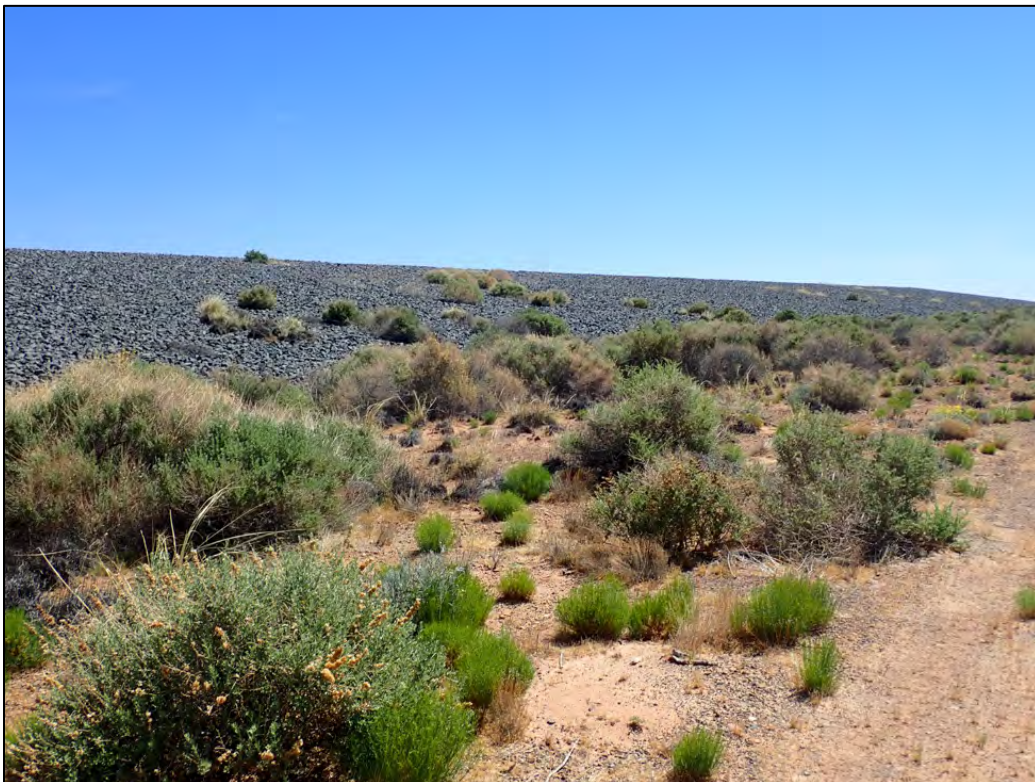
PL-8. Vegetation on South Slope of Disposal Cell
