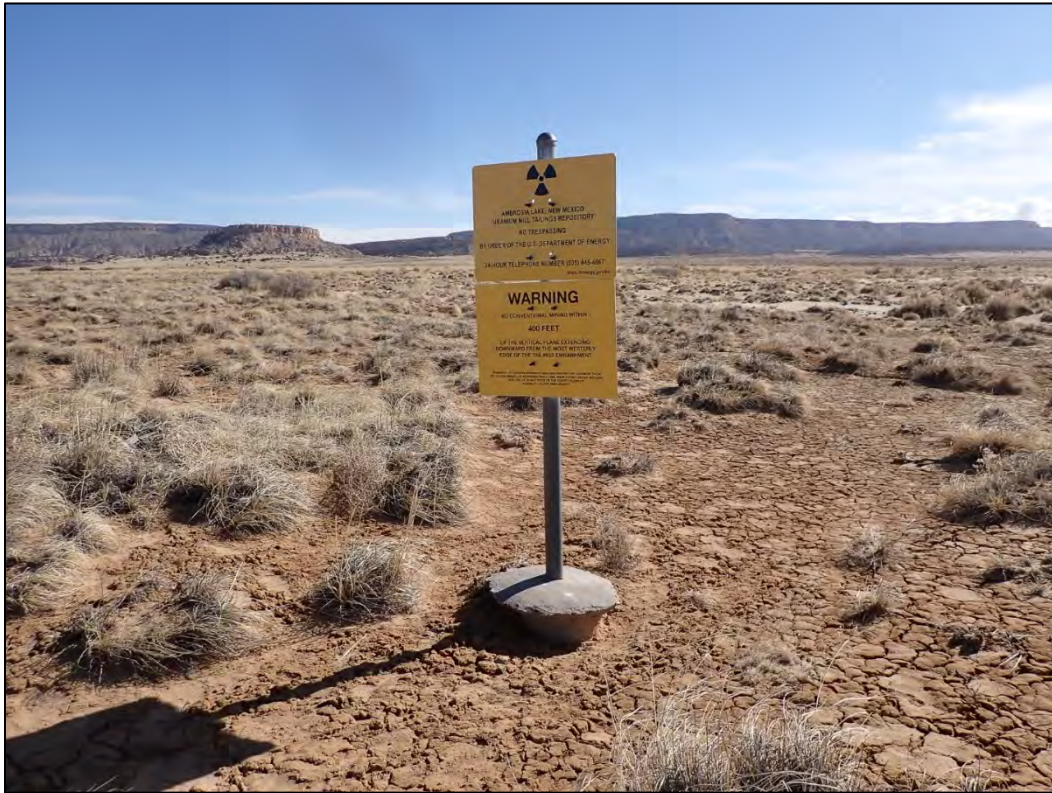
PL-3. Wind Erosion at Base of Perimeter Sign P12
