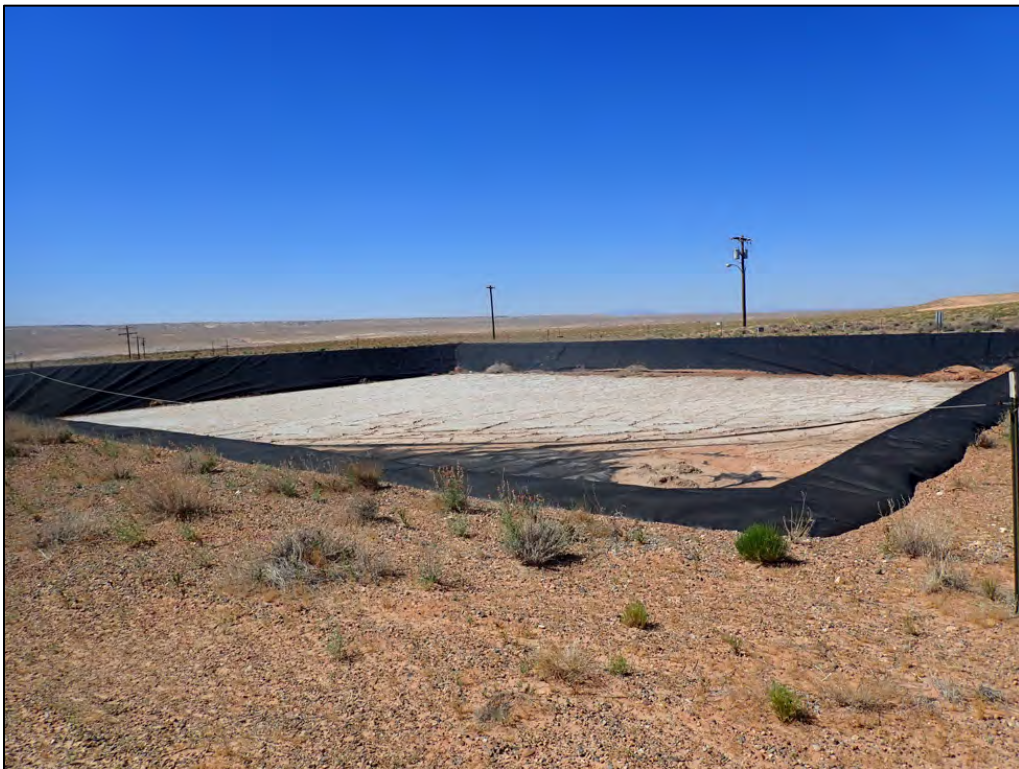
PL-10. Inactive Evaporation Pond
