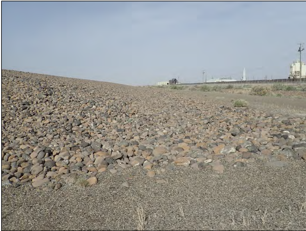
PL-5. Northern Cell Side Slope
