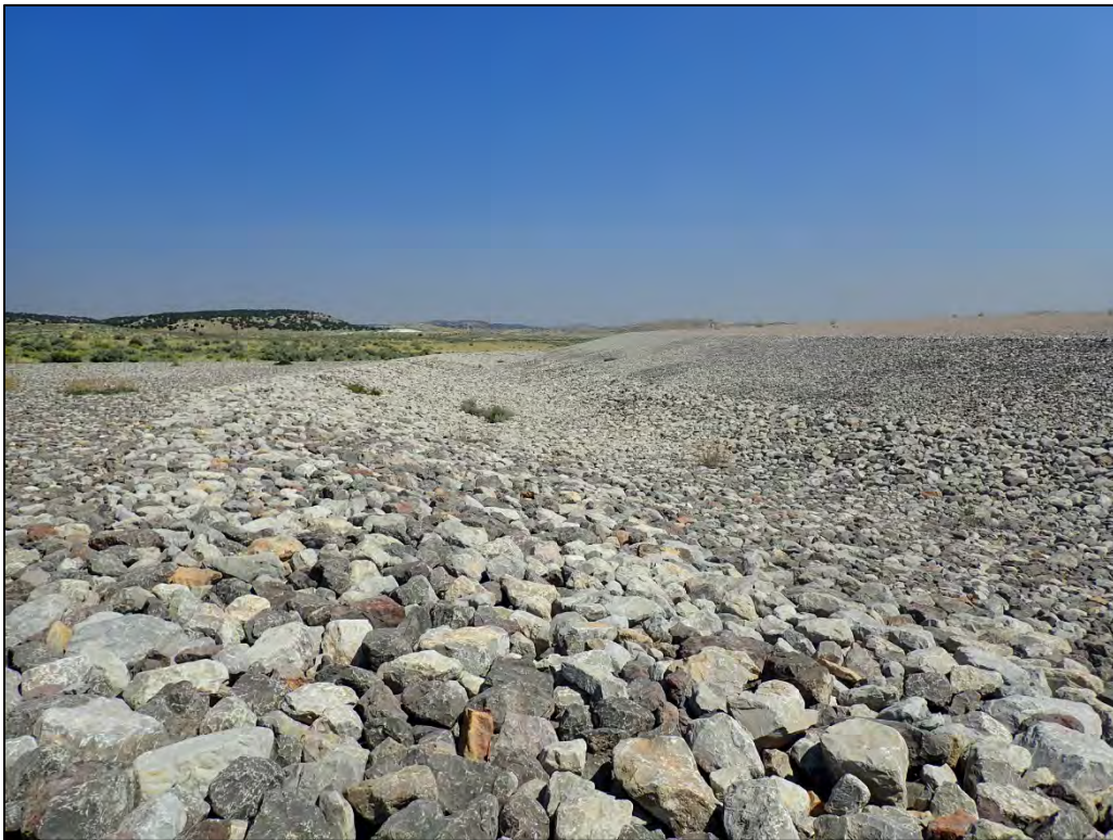
PL-10. Diversion Channel No. 1
