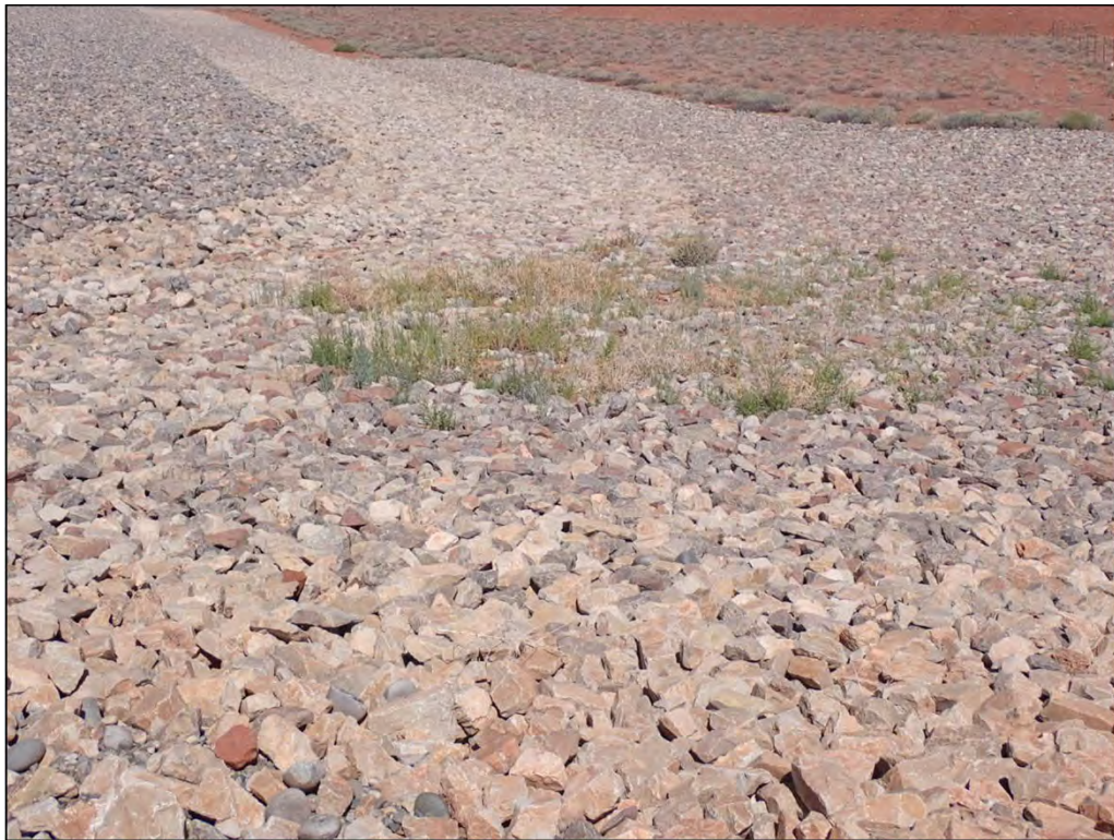
PL-8. Vegetation Growth in the West Diversion Channel
