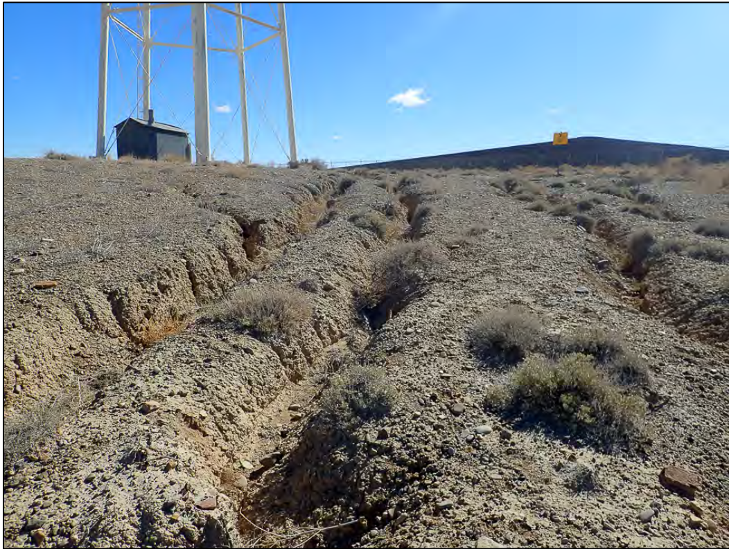
PL-13. Soil Erosion near Perimeter Sign P7
