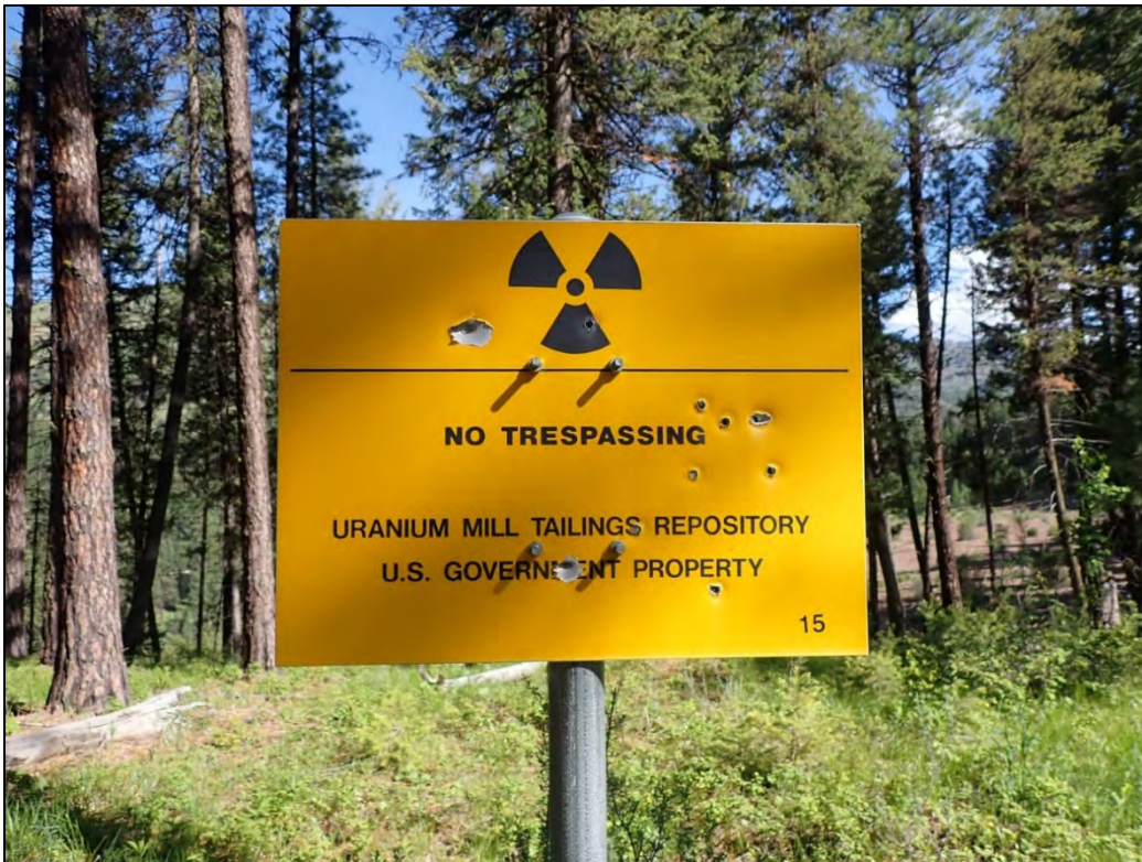
PL-2. Perimeter Sign P15 with Bullet Damage
