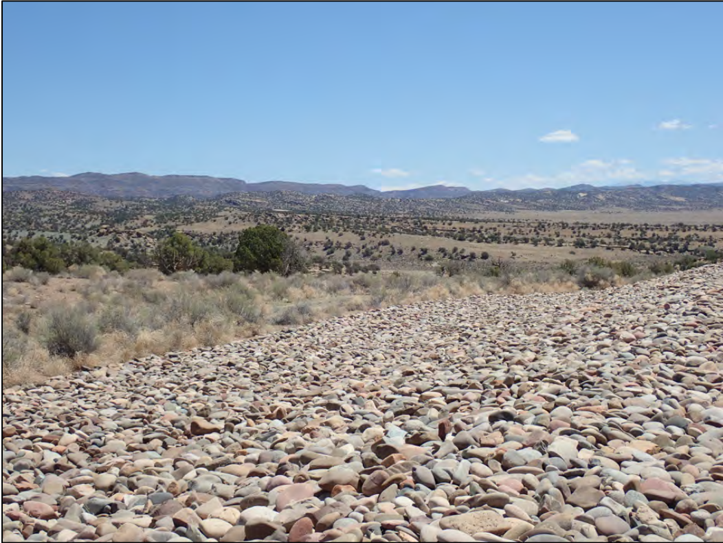
PL-5. Key Trench on East Side Slope
