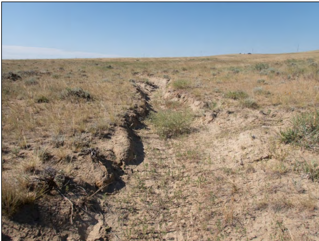
PL-6. Erosional Gully, Previously Unreported
