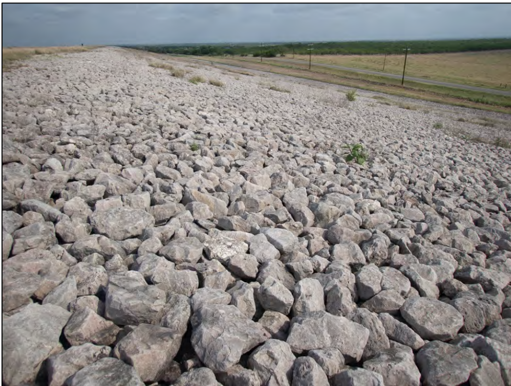
PL-8. Northeast Side Slope
