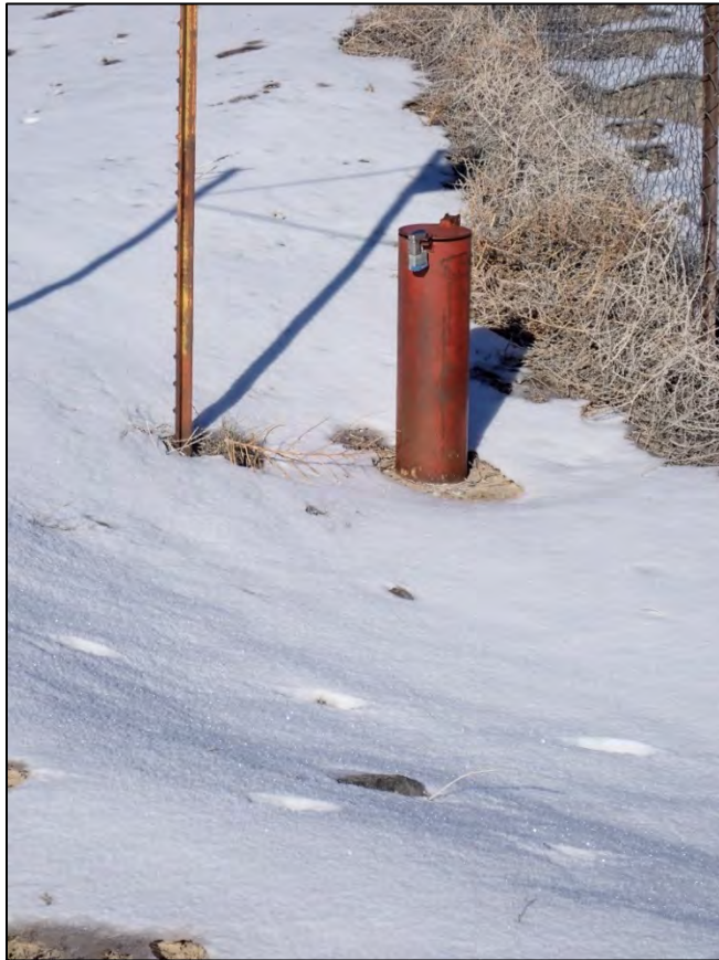
PL-7. Monitoring Well 0733
