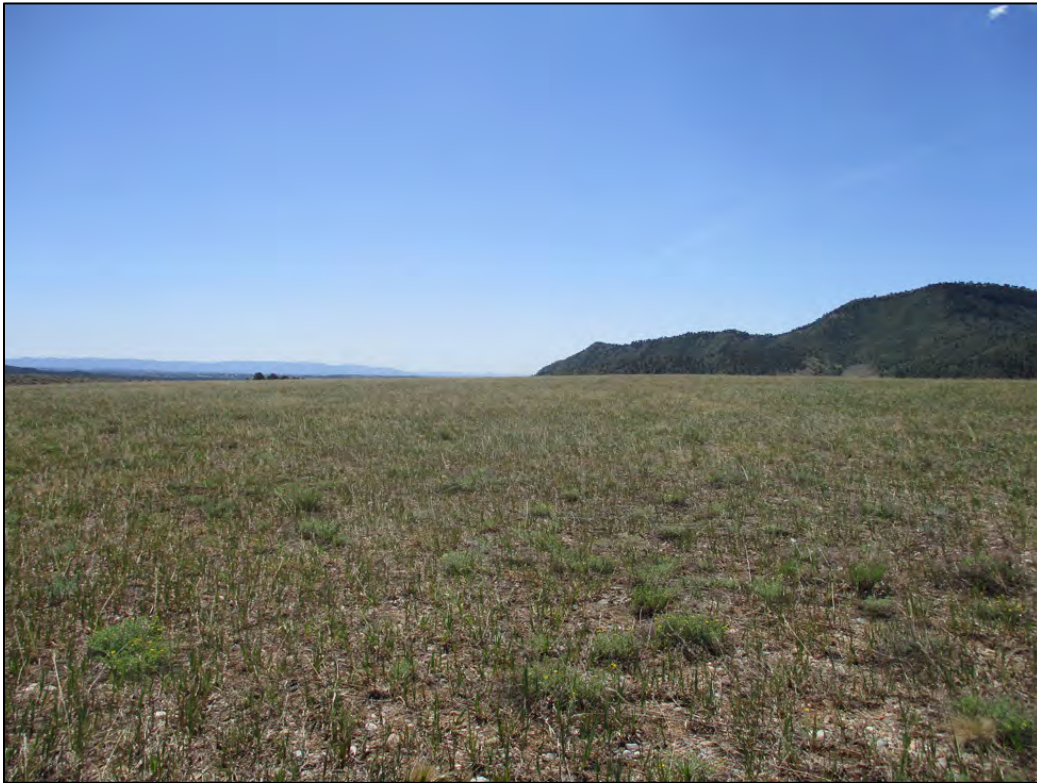
PL-5. Top of Disposal Cell, Looking Southeast
