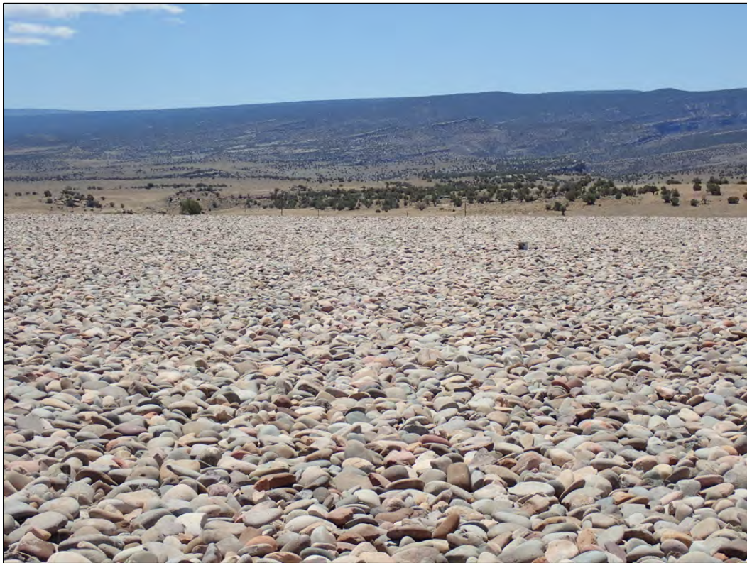
PL-4. Disposal Cell Top Slope
