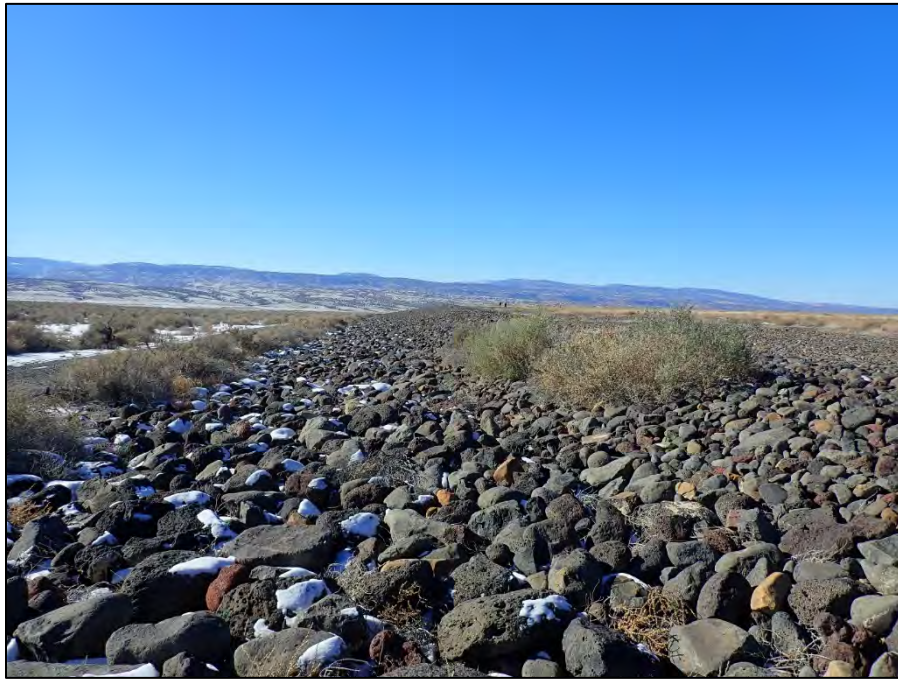
PL-8. South Side Slope of Disposal Cell
