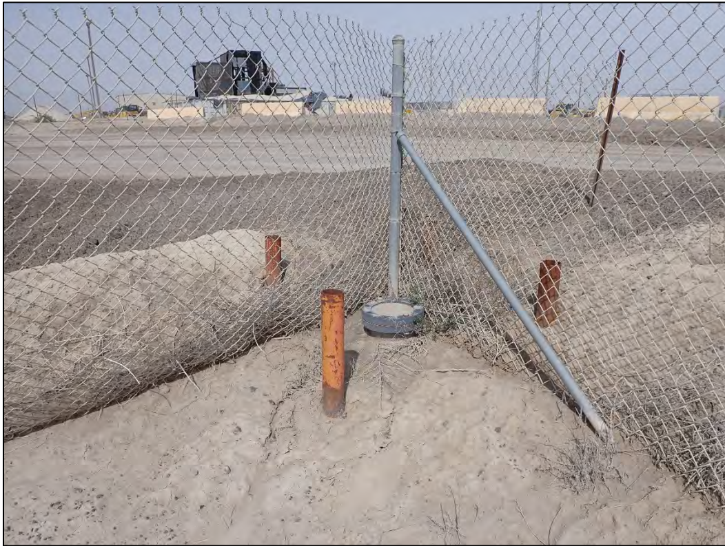
PL-3. Boundary Monument BM-1 with Protective Cover and Nearby Bollards
