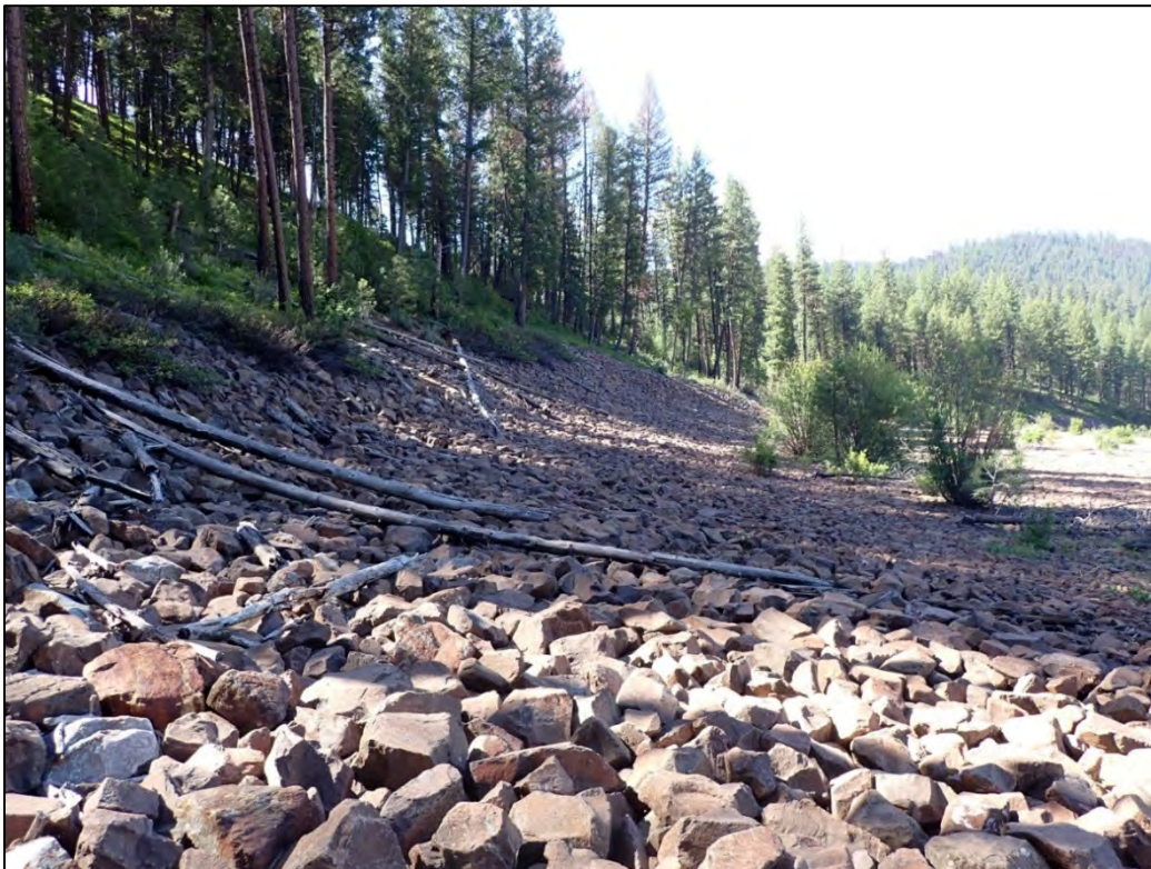
PL-6. Disposal Cell Apron on Eastern Side
