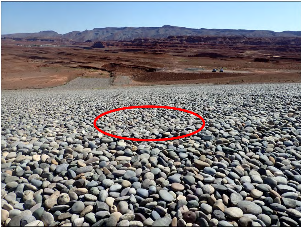
PL-6. Depression Feature on the Northeast Side Slope
