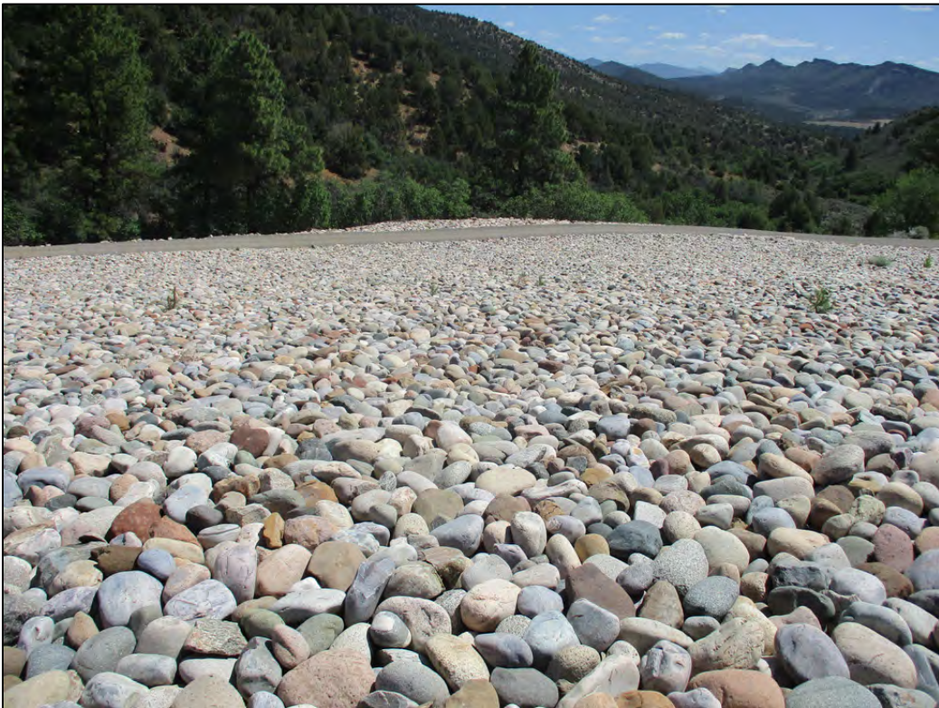
PL-8. Young Ponderosa Pines in Riprap Along North Side Slope
