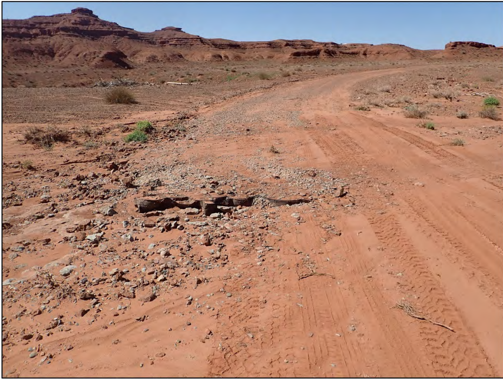
PL-1. Access Road with Minor Erosion
