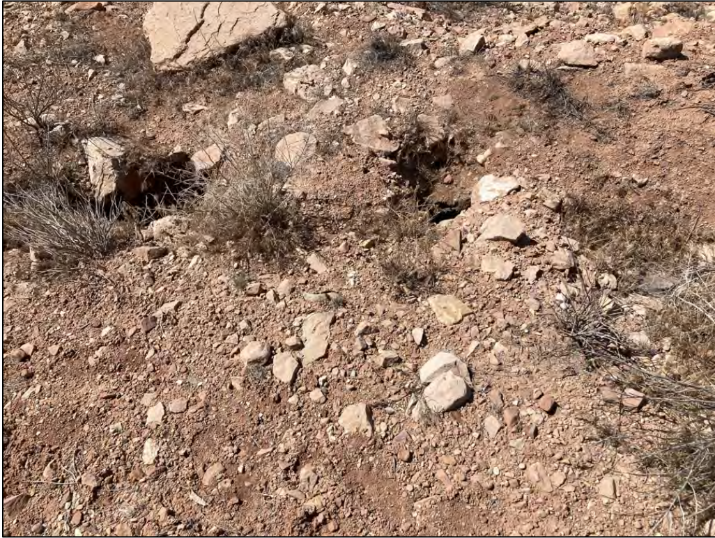
PL-7. Erosional Channeling on Slope North of Disposal Cell
