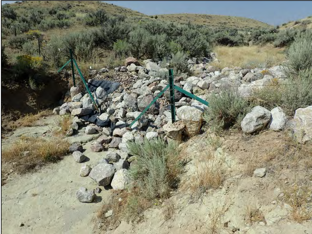
PL-11. Exposed Geofabric in Diversion Channel No. 1
