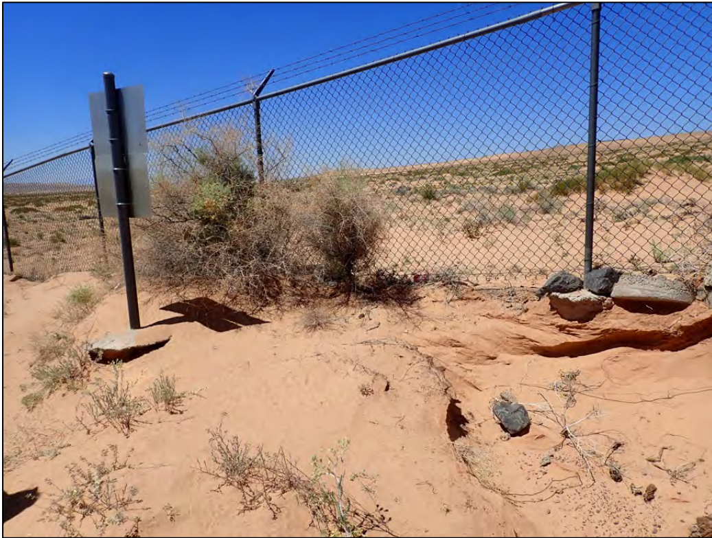
PL-3. Vegetation and Debris on Fence near Perimeter Sign P9
