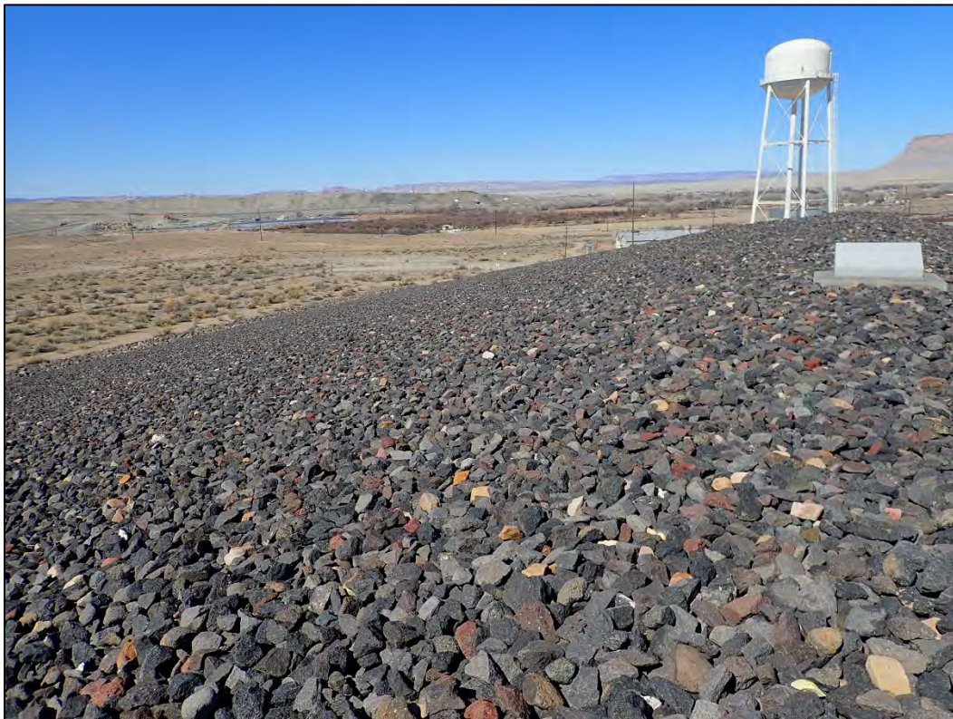
PL-4. Disposal Cell Southwest Side Slope and Site Marker SMK-2
