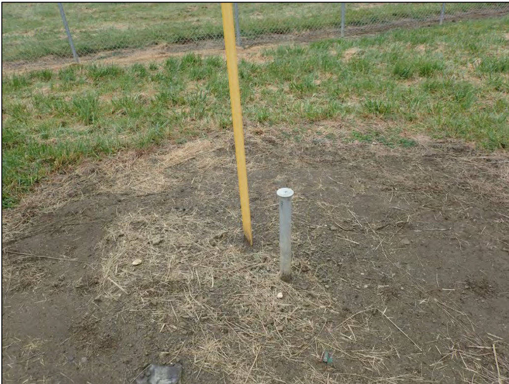
PL-6. Erosion Control Marker 3
