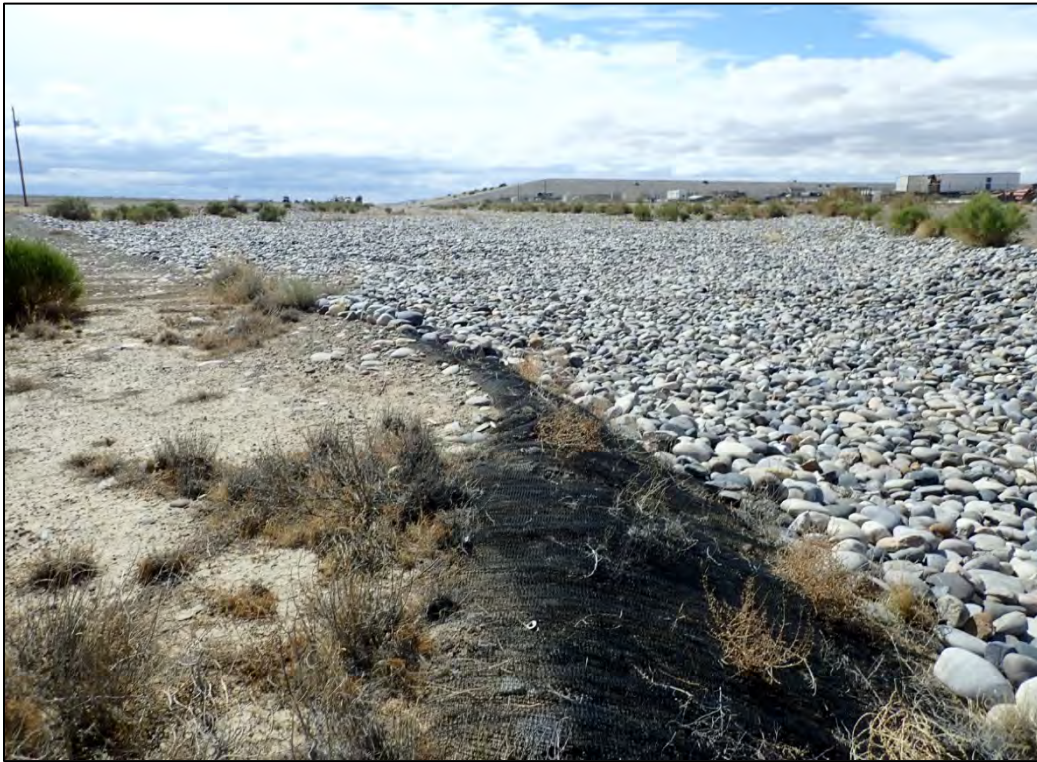
PL-9. Northwest Drainage Channel
