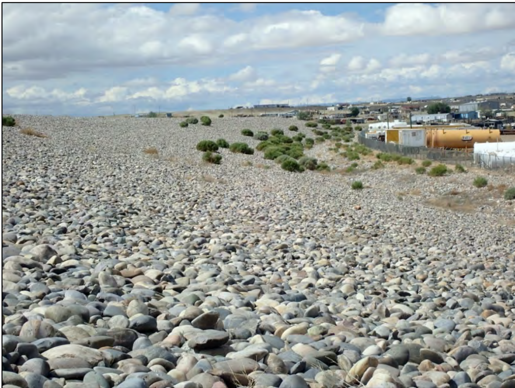
PL-8. West Side Slope of Disposal Cell
