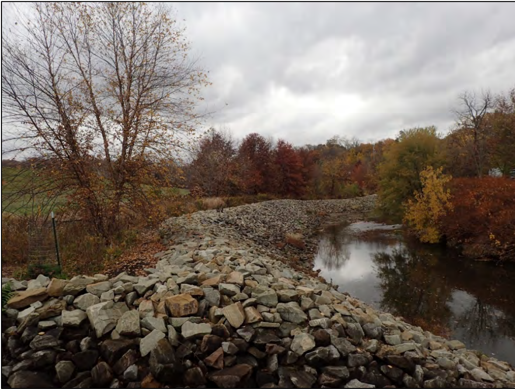
PL-10. Riprap-Armored Streambank
