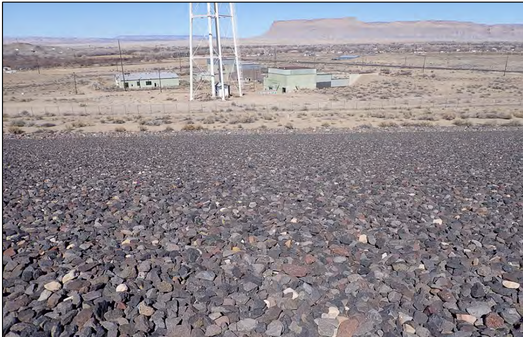
PL-14. Northwest Disposal Cell Side Slope
