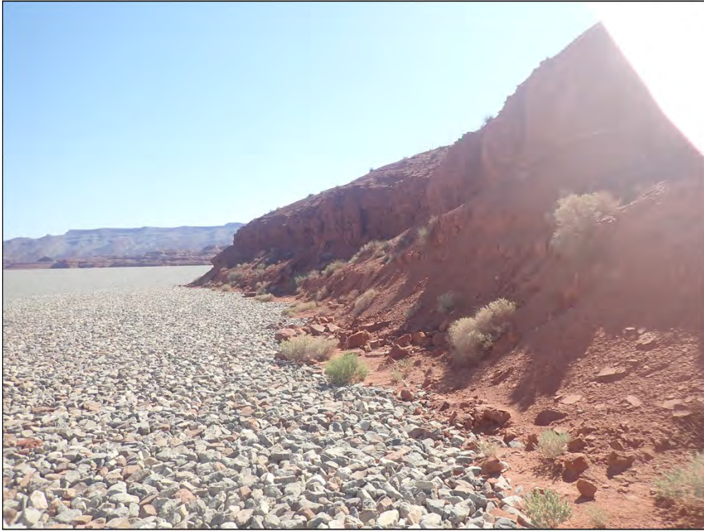
PL-7. Sloughing Rock Along the South Apron
