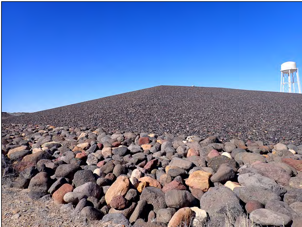
PL-8. Northeast Side Slope of Disposal Cell
