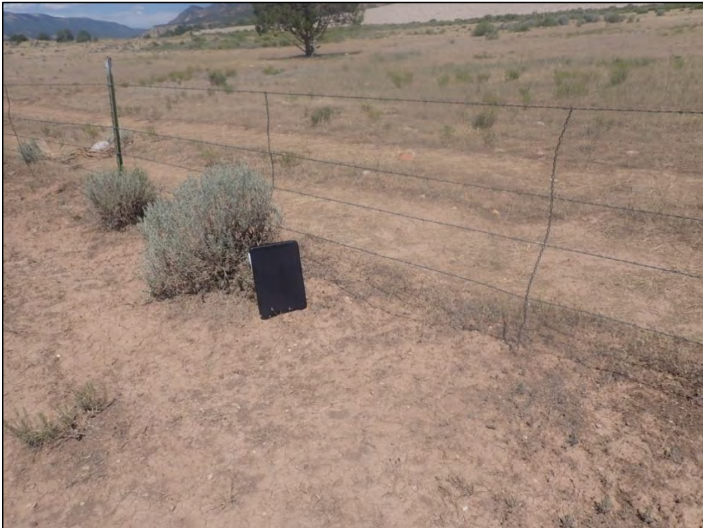
PL-10. Signs of Animal Burrowing Under Fence
