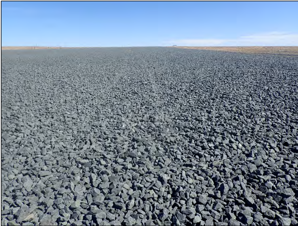
PL-7. Parallel Tracks Visible on Top of Disposal Cell
