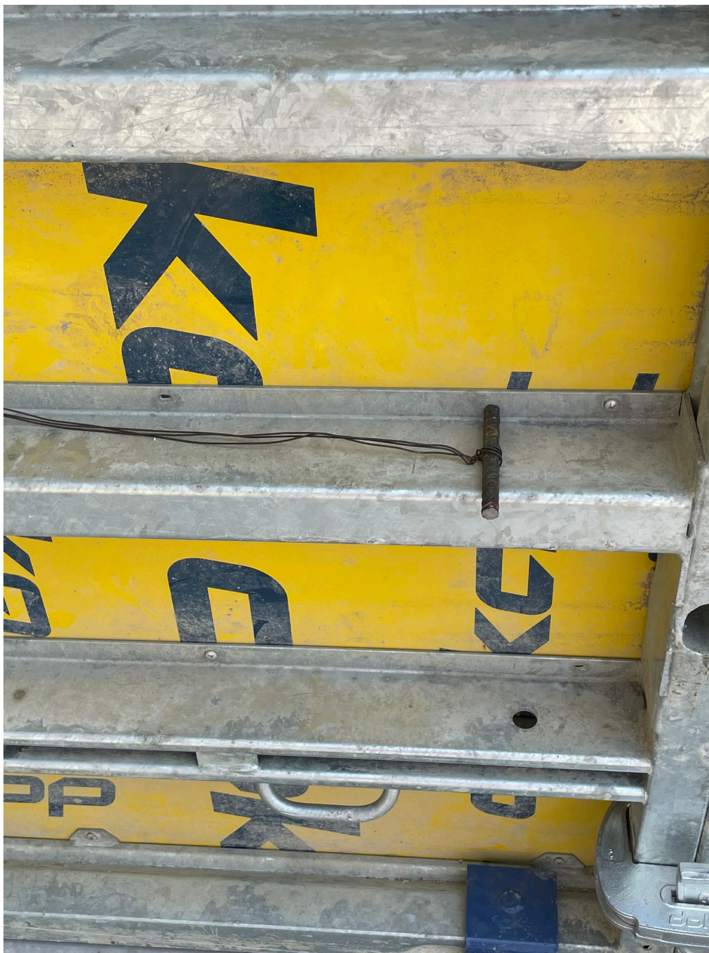
Figure 2-4. Example of Rebar Tie
