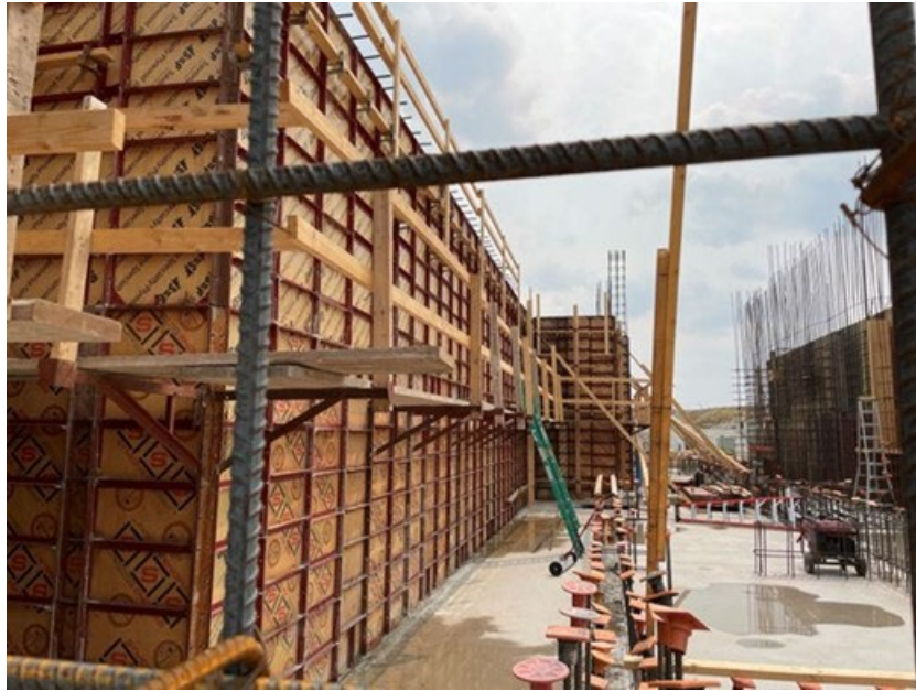
Figure 3-7. Scaffolding and Ladders on Previously Installed Symons Formwork
