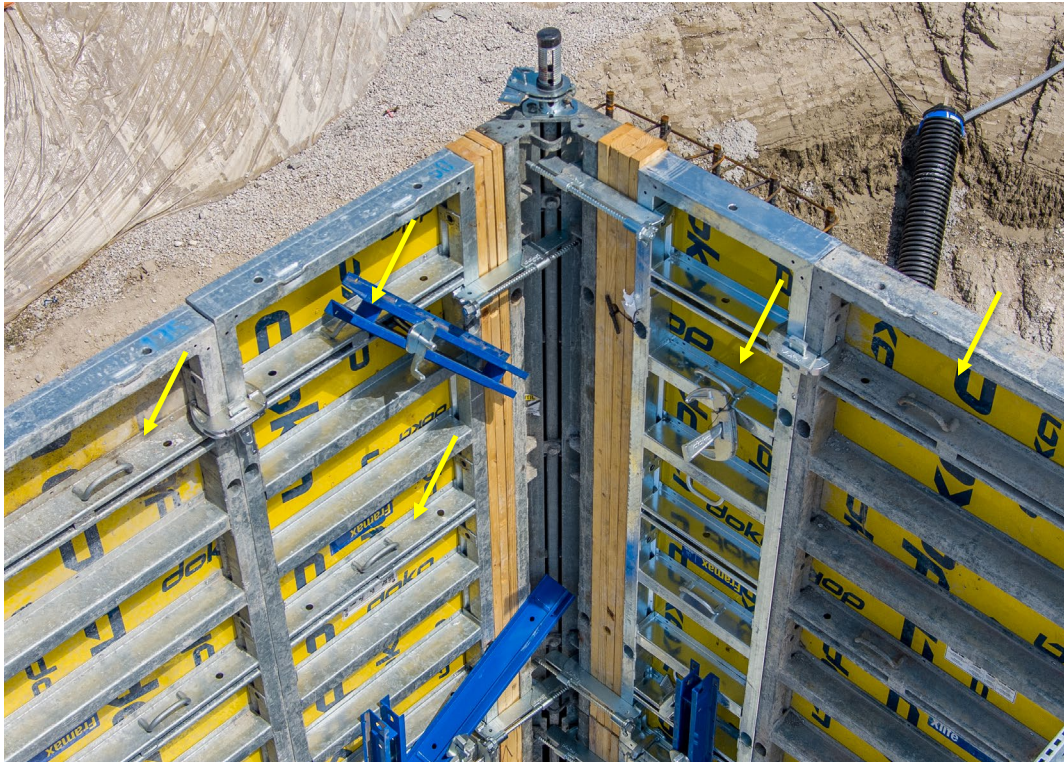
Figure 3-2. Doka Integrated Handles (Northwest Corner)
