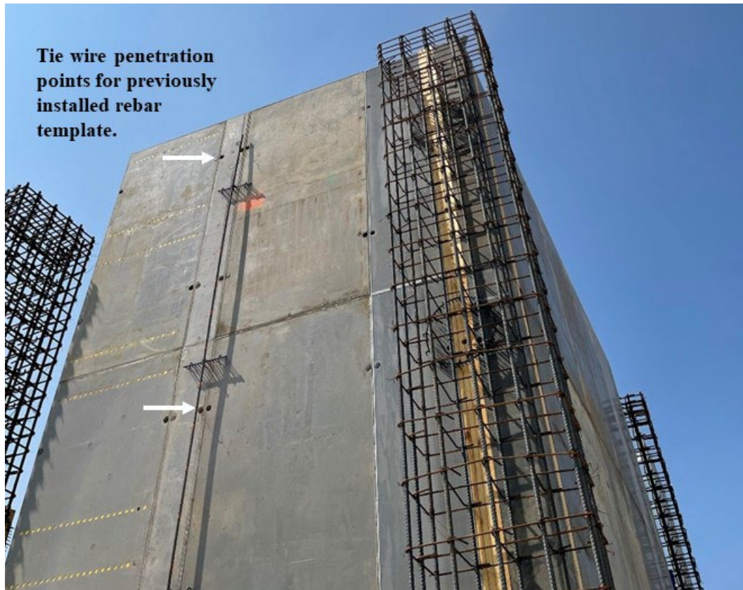
Figure 2-3. North Side of Doka Form Wall with Installed Template Bar and Tie Wire Penetration Points
