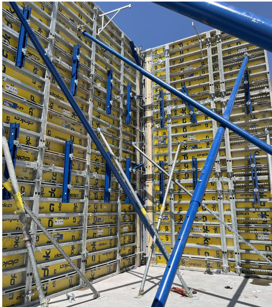
Figure 2-1. Northwest Corner of Doka Formwork
