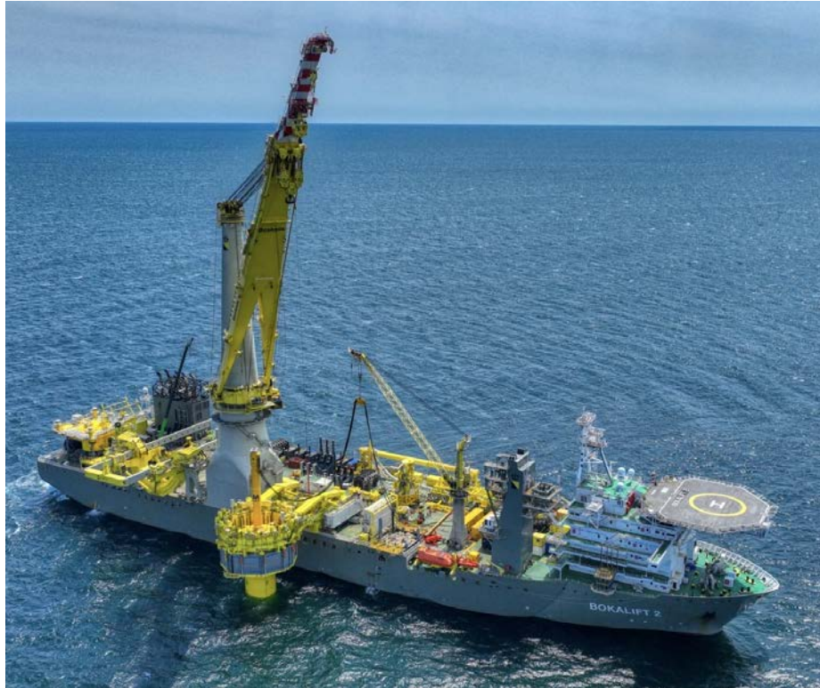
Installation of first monopile foundation at South Fork Wind Farm. Photo courtesy of South Fork/Boskalis
