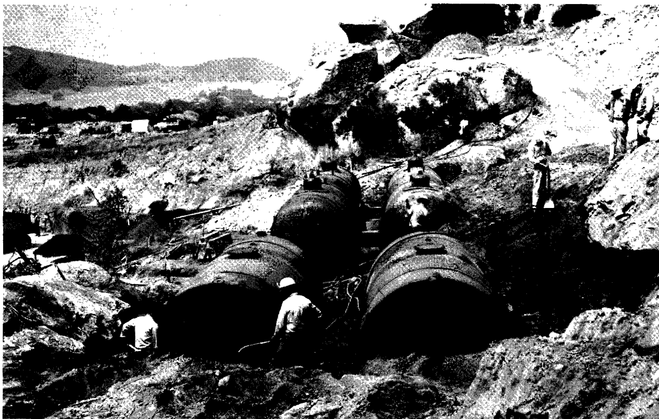
Figure 11. Arrangement of R/A Liquid Waste and Vent Systems Tanks (Construction Phase)
