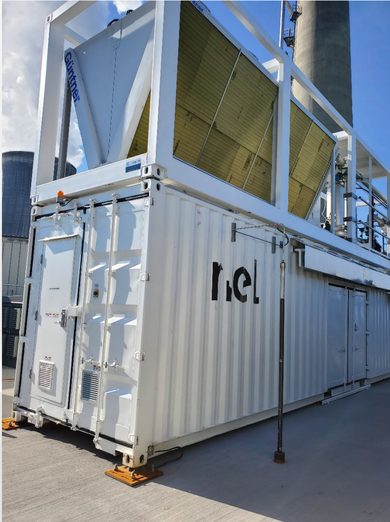
Electrolyzer and cooling unit to left Compressor below
