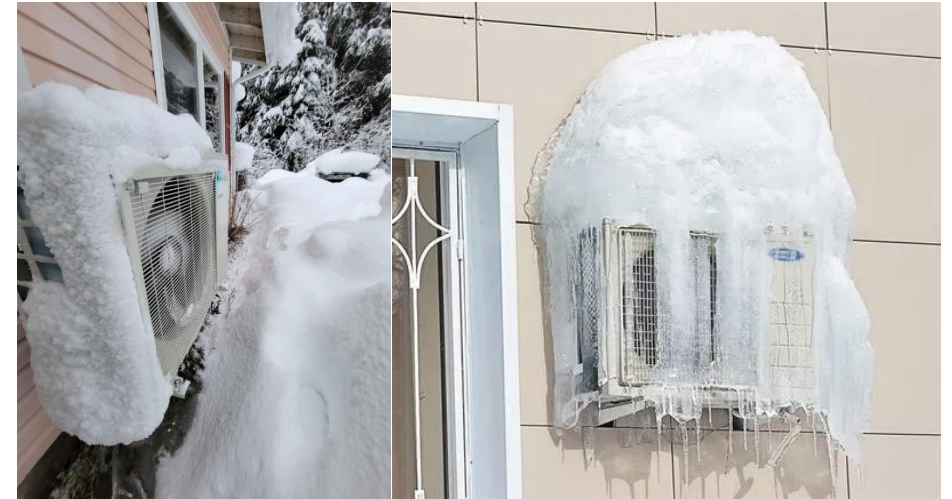
Frost/ice buildup in the outdoor coils of cold climate heat pumps in Alaska.
