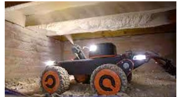
Q-Bot for crawlspace SPF install
