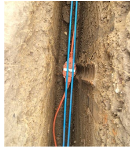
F/O Deployed in Trench
