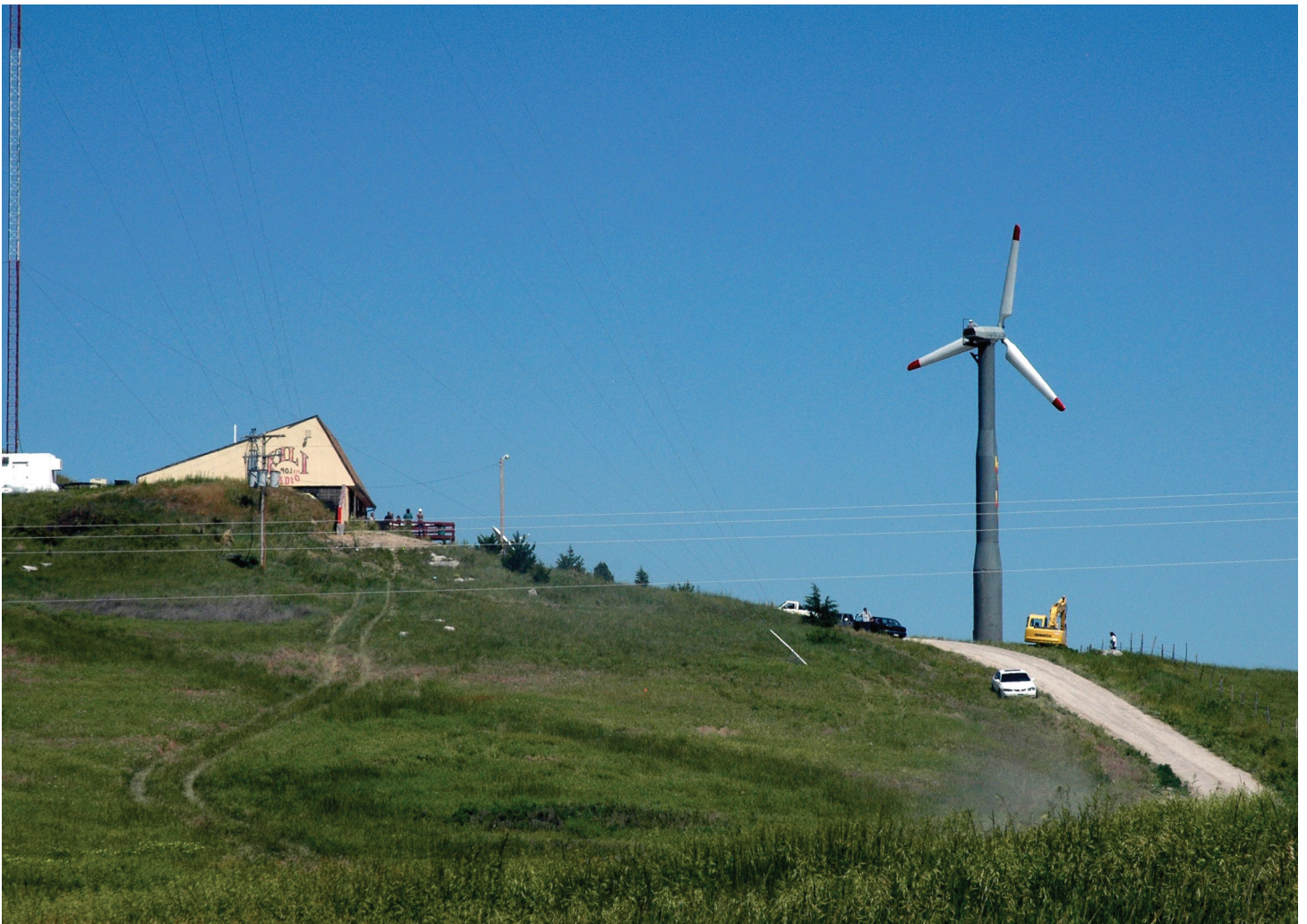
The Lakota Nation installed a 65-kW Nordtank turbine that annually supplies 120 MWh of power to KILLI, the Pine Ridge Reservation radio station known as the voice of the Lakota Nation in South Dakota. Photo by Bob Gough, NREL 16258
