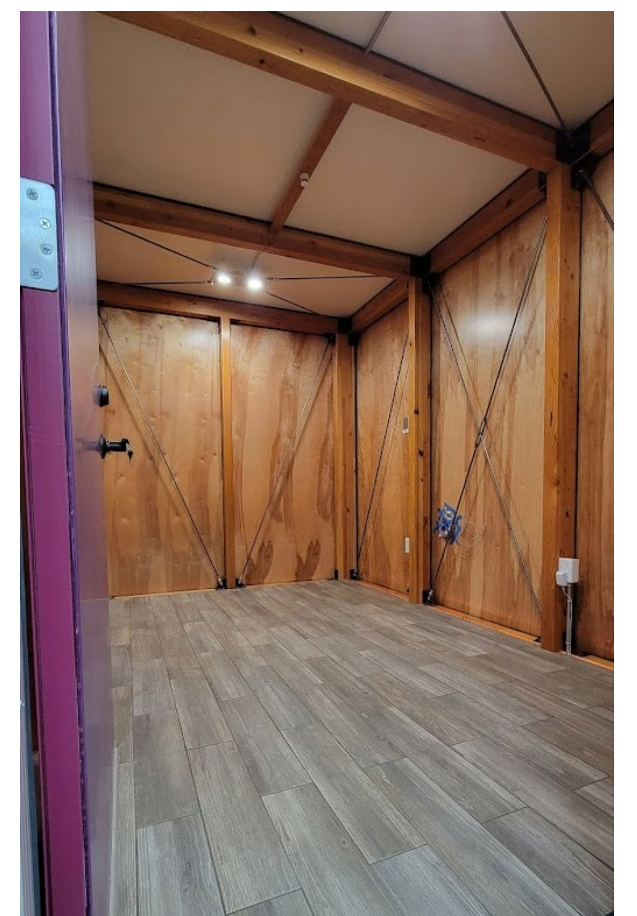
The structural frame is made with standard glulam lumber, each 4' x 8'. Adaptable composite panel has four 1-in. thick 2' x 4' fiberglass-core VIPs, and the basic building system provides aesthetics. Photos by Stacey Fritz, NREL
