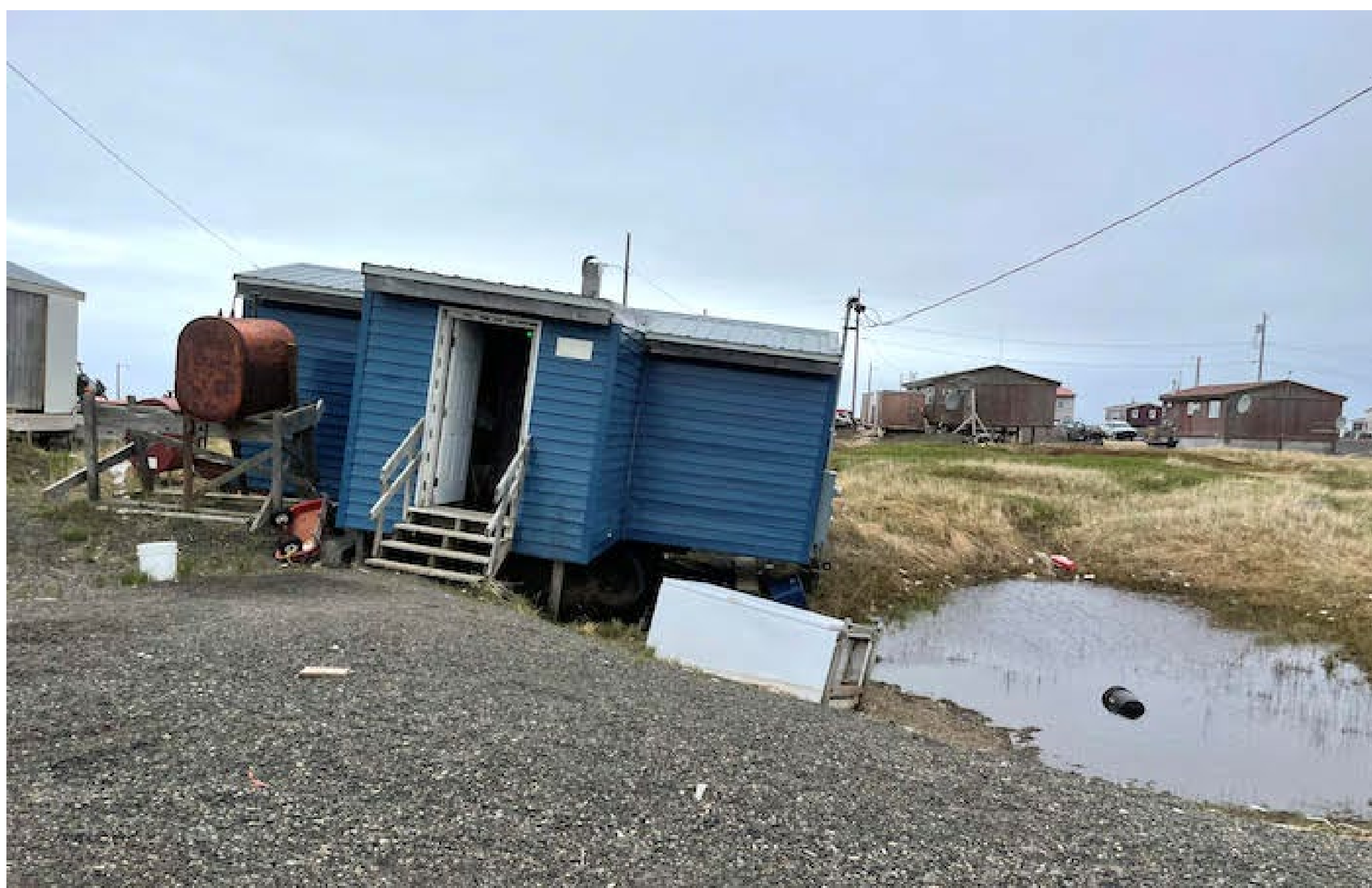
Permafrost subsidence-damaged home in Pt. Lay, AK. Photo from Ben Jones, UAF
