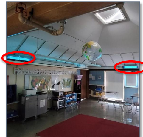
Left: "Upper-room" GUV installation at Cambridge Friends School, Cambridge, MA Right: "Whole-room" GUV installation at Hartsfield-Jackson Atlanta Airport
