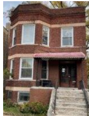
2-4 flat Pre-1942 Masonry/brick construction Comprehensive
