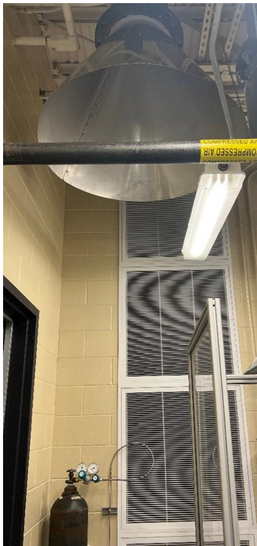
Dilution tunnel intake
