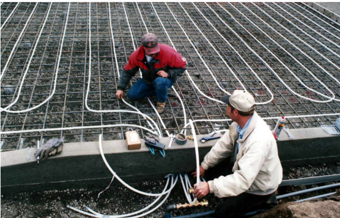
Installation of snowmelt tubing in slurry backfill under sidewalks in Klamath Falls, OR, which the city uses to melt snow on more than 50,000 square feet of sidewalks and crosswalks as part of its district heating system. Photo courtesy Geo-Heat Center / NREL pix 08832.
