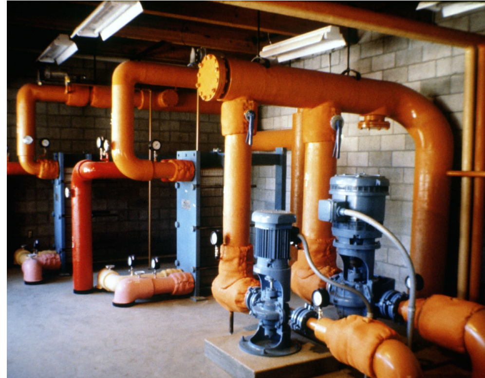
Heat exchangers and circulation pumps in Klamath Falls, OR, district geothermal system. Photo courtesy Geo-Heat Center / NREL pix 03694
