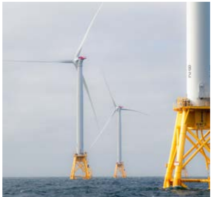
The Block Island Wind Farm, the first U.S. offshore wind farm, represents the launch of an industry that has the potential to contribute significantly to a reliable, stable, and affordable energy mix. Photo by Dennis Schroeder, NREL 41193
