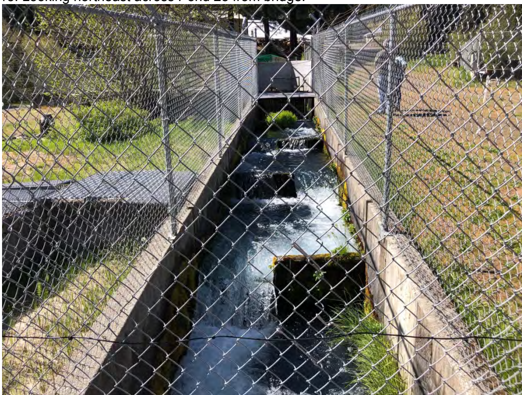
Photo 16. Looking southwest along fish ladder that flows out of the hatchery pond.
