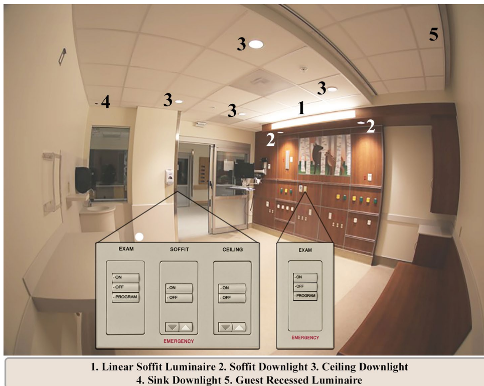
Figure 2. NICU Patient Room Prior to Occupancy. The white-tunable luminaires connected to the LCS are all operating in this photo. The infant bed (not pictured) is placed perpendicular to the headwall, under the soffit.
