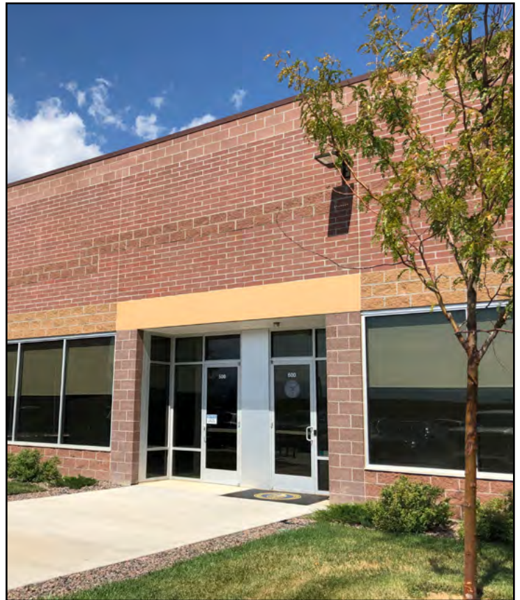
DOE Legacy Management Operations Center in Westminster, Colorado, earned the EPA ENERGY STAR Tenant Space designation.
