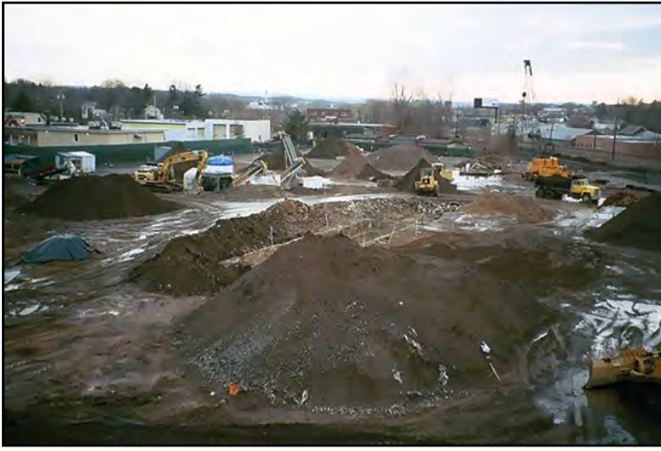
The former NL Industries Inc. plant during remediation.
