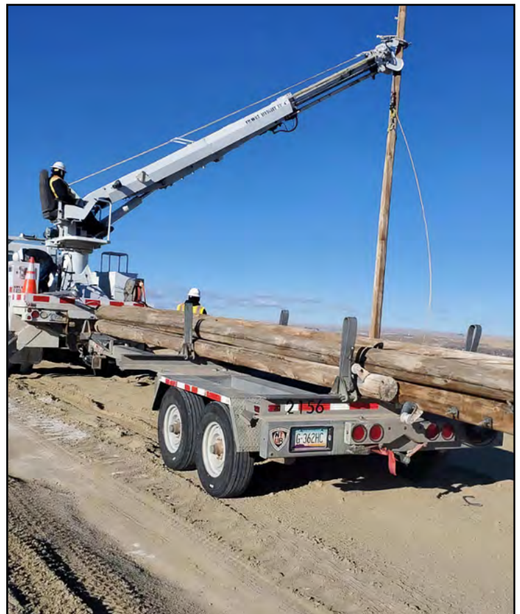
Navajo Tribal Utility Authority workers remove power poles.
