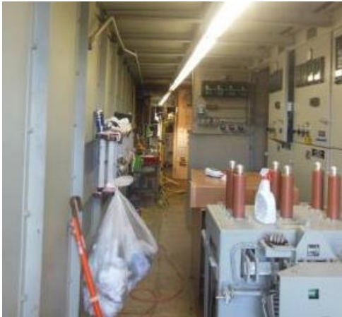
Figure 3-2. This photo shows the front of de-energized Bus A. Note the one air breaker on the floor, as well as a bench, trash, and extension cord, and scattered tools.
