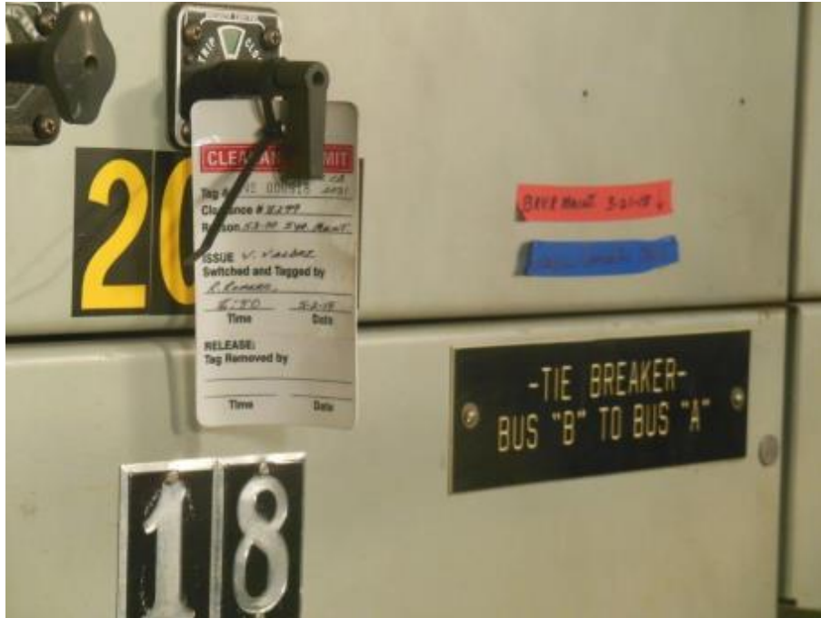
Figure. 2-3. The Clearance Tag hangs from the cubicle 18 tiebreaker.
