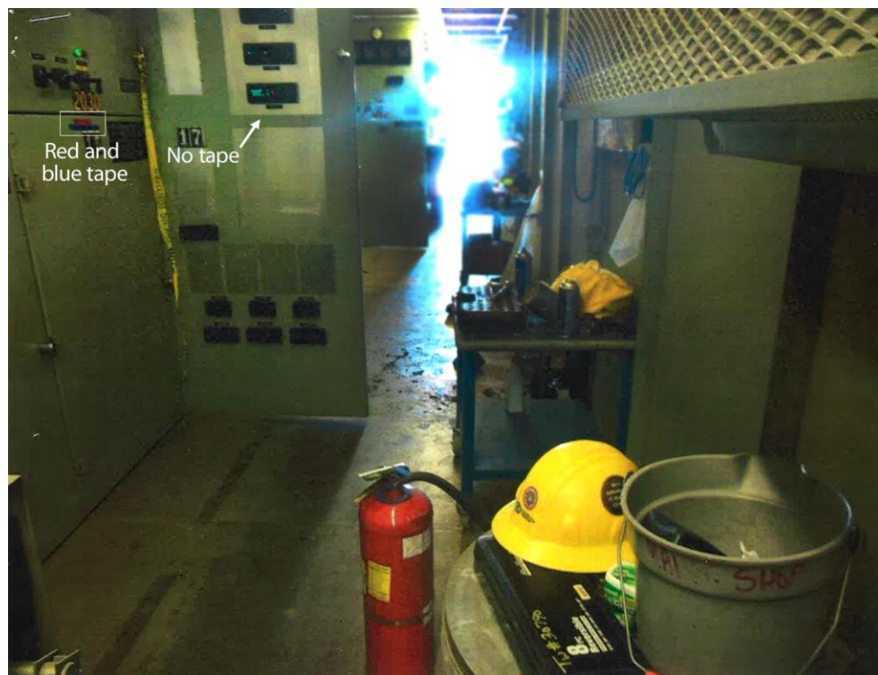
Figure. 3-4. No tape was found on cubicle 17. Note the red and blue tape on the adjacent cubicle.
