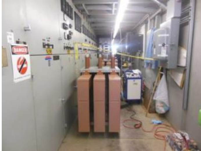
Figure 3-1. This photo shows the area in front of energized Bus B and Bus C, both of which power the LANSCE area. Note how close the breakers under test were set to the operating equipment. There is an open cubicle door on the operating area. The blue device is the hi-pot test set. The area is so crowded that it almost blocks the east side exit door.
