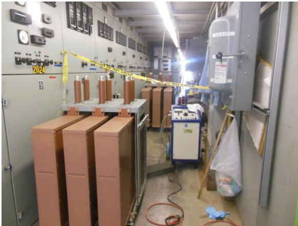
Figure. 3-5. Yellow caution tape was used as a barrier for hi-pot testing.
