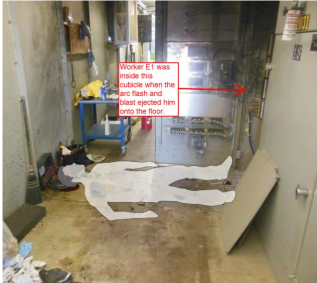
Figure. 2-10. Position of E1 after the arc-flash event.
