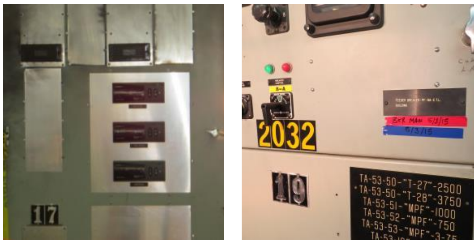
Figure 3-6. Cubicle 19 showing both the breaker testing and cleaning is complete, in contrast to Cubicle 17 with no tape on Sunday, even though Cubicle 17 is on a re-energized bus.
