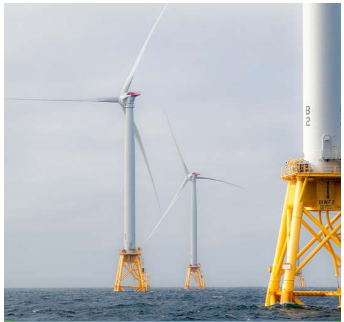
The Block Island Wind Farm, the first U.S. offshore wind farm, represents the launch of an industry that has the potential to contribute significantly to a reliable, stable, and affordable energy mix. Photo by Dennis Schroeder, NREL 41193
