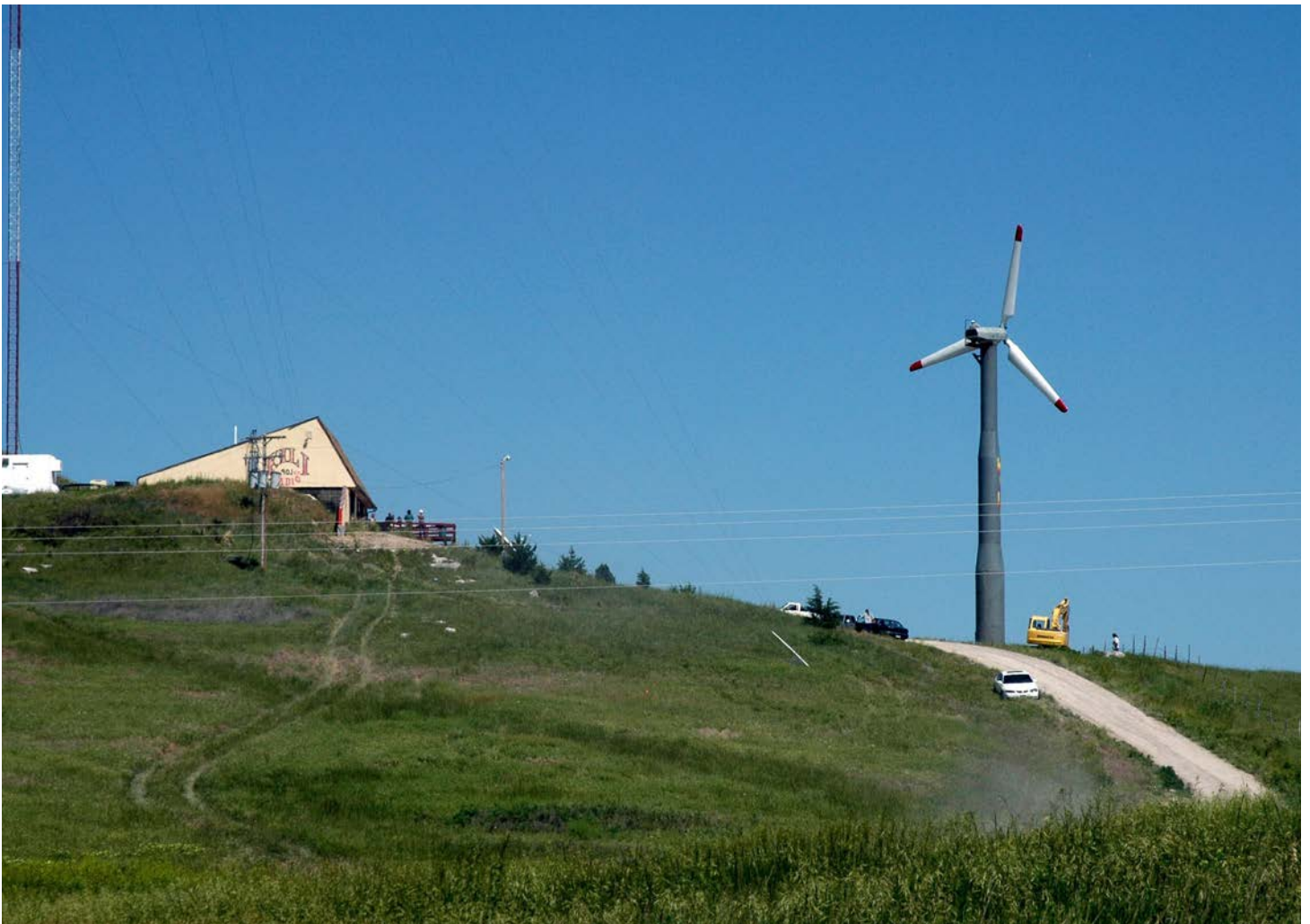
The Lakota Nation installed a 65-kW Nordtank turbine that annually supplies 120 MWh of power to KILLI, the Pine Ridge Reservation radio station known as the voice of the Lakota Nation in South Dakota. Photo by Bob Gough, NREL 16258
