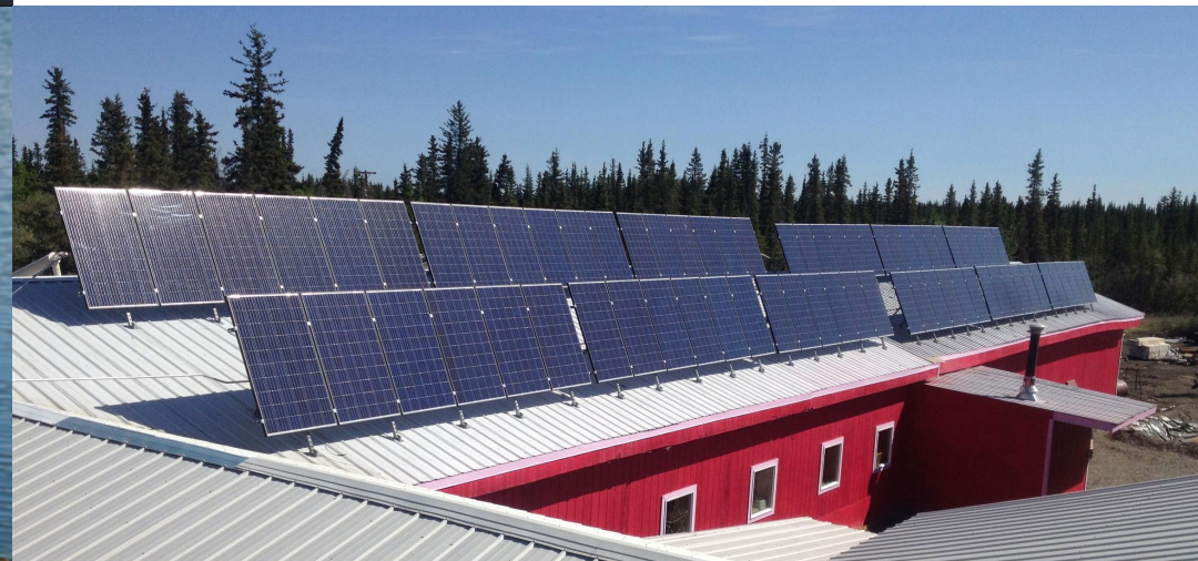
Photovoltaic array on the Tribal Hall in Fort Yukon, Alaska. Photo from Dave Pelunis-Messier, Tanana Chiefs Conference
