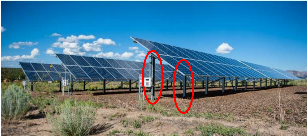
Figure 5. A system using front and back support posts (circled)
