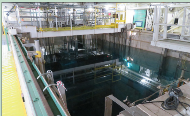
This 27-foot pool in Building 3010 housed irradiated items from the former research reactor.
