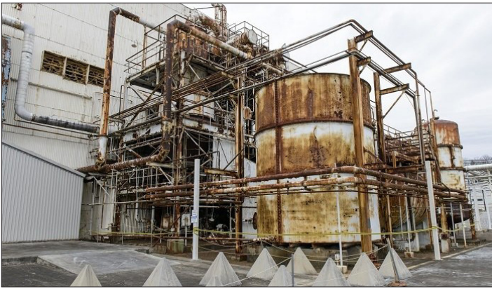
The exterior of the column exchange processing structure on the east side of the Alpha-4 facility at the Y-12 National Security Complex. Removing this deteriorated equipment will eliminate risks and move Alpha-4 closer to demolition.
