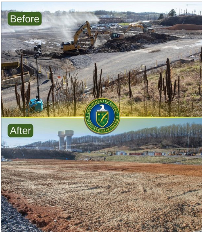
Oak Ridge workers spent much of 2022 tearing up and removing building slabs left behind from the Biology Complex demolition, as shown at top.
