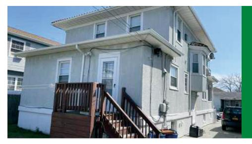
The low-sloped hip-roof design has helped the home survive the hurricanes that travel up the Atlantic Coast and may explain why the original clay tile roofing is still intact. The project team decided to wrap the stucco in taped rigid foam then install vinyl siding over top to encase the lead paint and provide a continuous air, water, and thermal barrier around the home.
