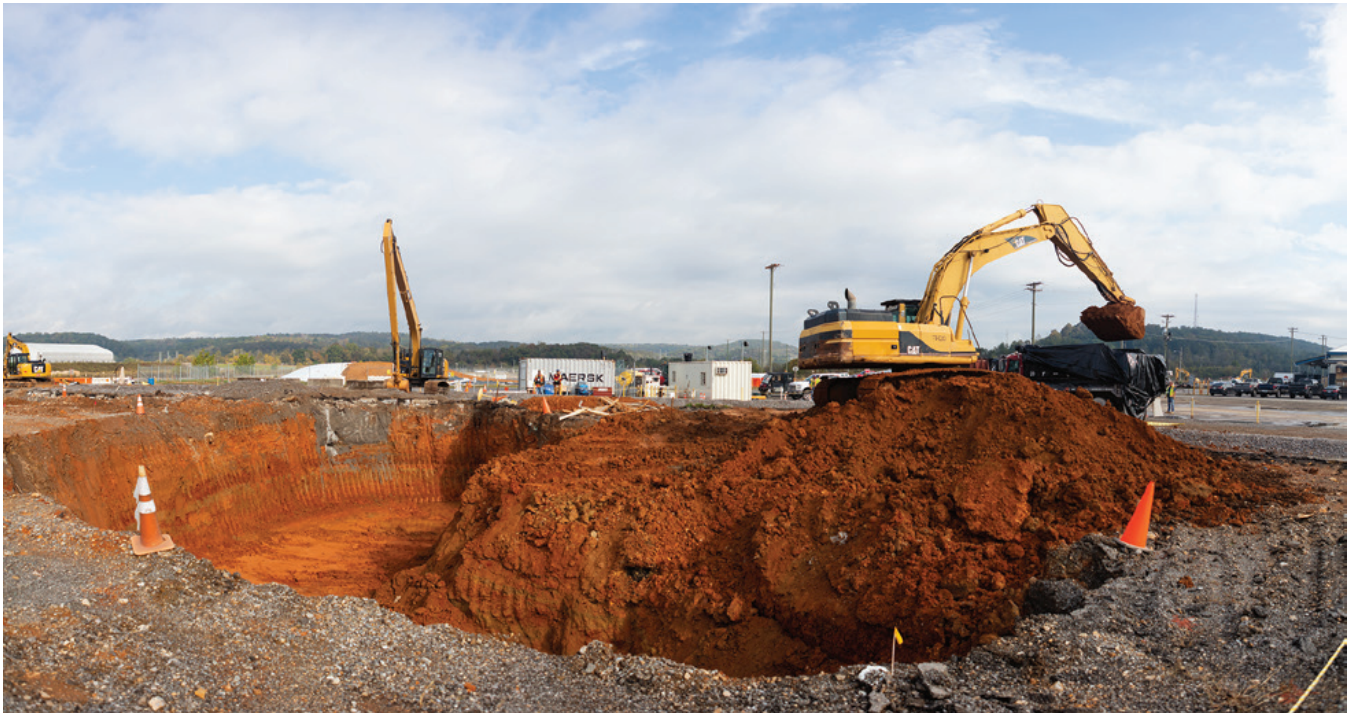
Remediation at EU-25 involved removing building slabs and underlying soil.
