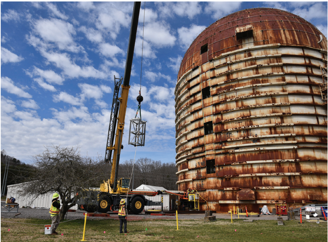
Installation of transport platform cart system
