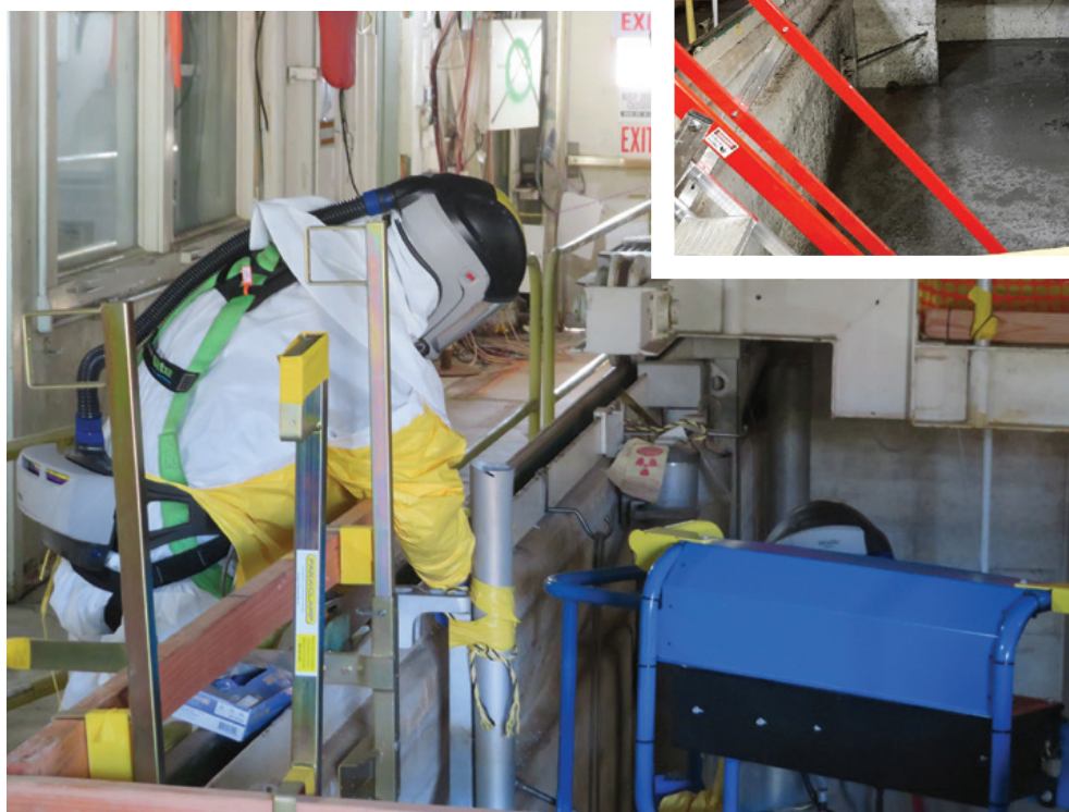
A worker samples the pool wall in the Bulk Shielding Reactor (left). Above, the pool is being filled with a concrete mixture after components were removed and the pool drained.
