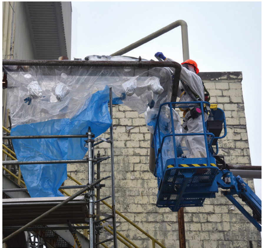
Workers wrap pipes at the Low Intensity Test Reactor as part of deactivation activities.
