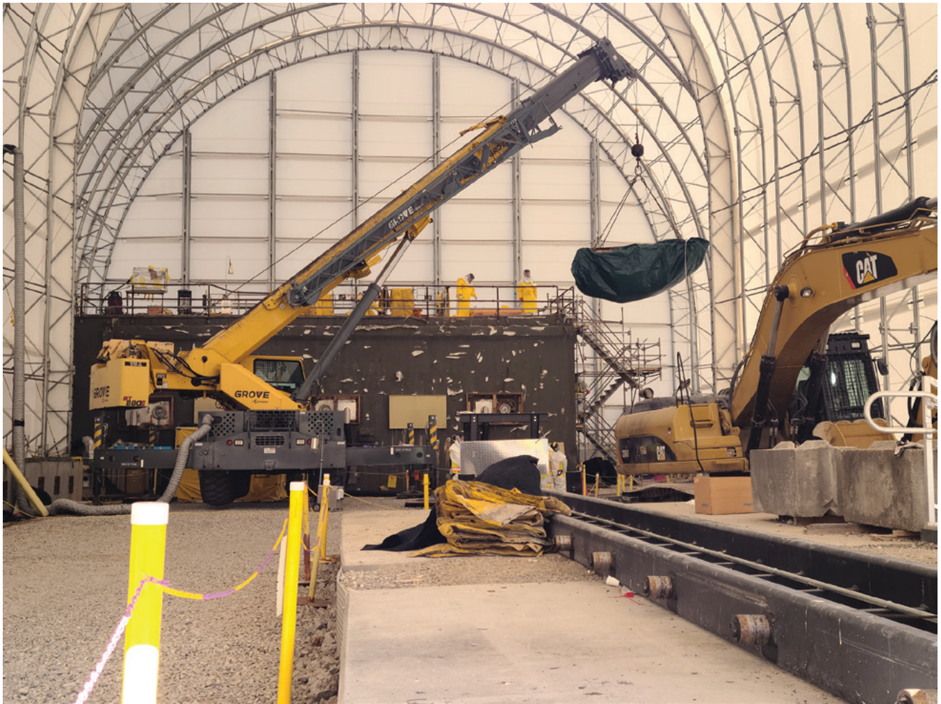
Workers remove sections of the hot cell roofing in order to access and characterize the structure.
