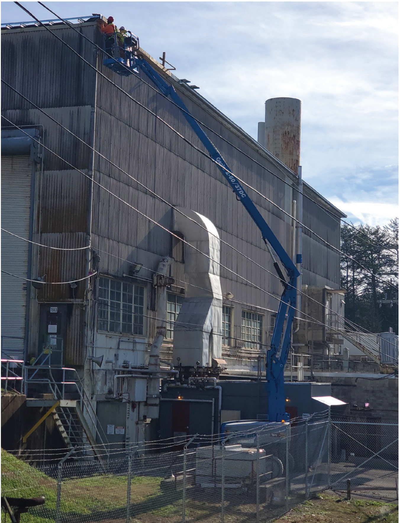
Workers install new roofing over the MSRE high bay to keep key systems protected.
