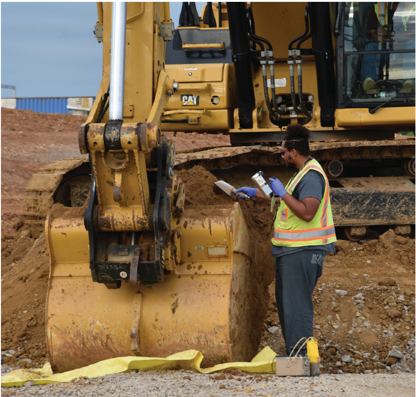
A worker checks for radioactivity levels in soil excavated at EU-21.
