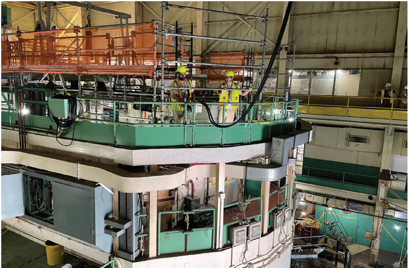
Workers wrap pipes at the Low Intensity Test Reactor as part of deactivation activities.
