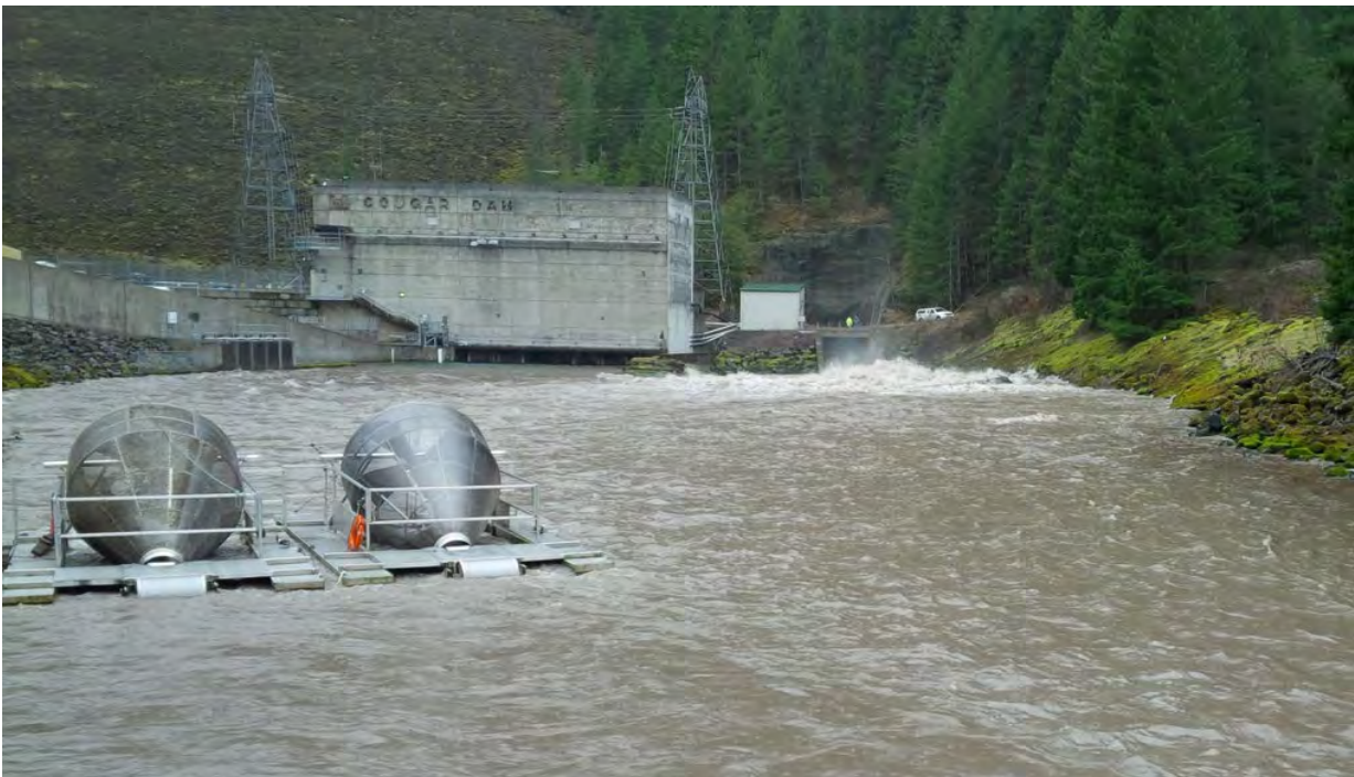
Figure ES- 26. Downstream view of Cougar diversion tunnel in action in 2016
