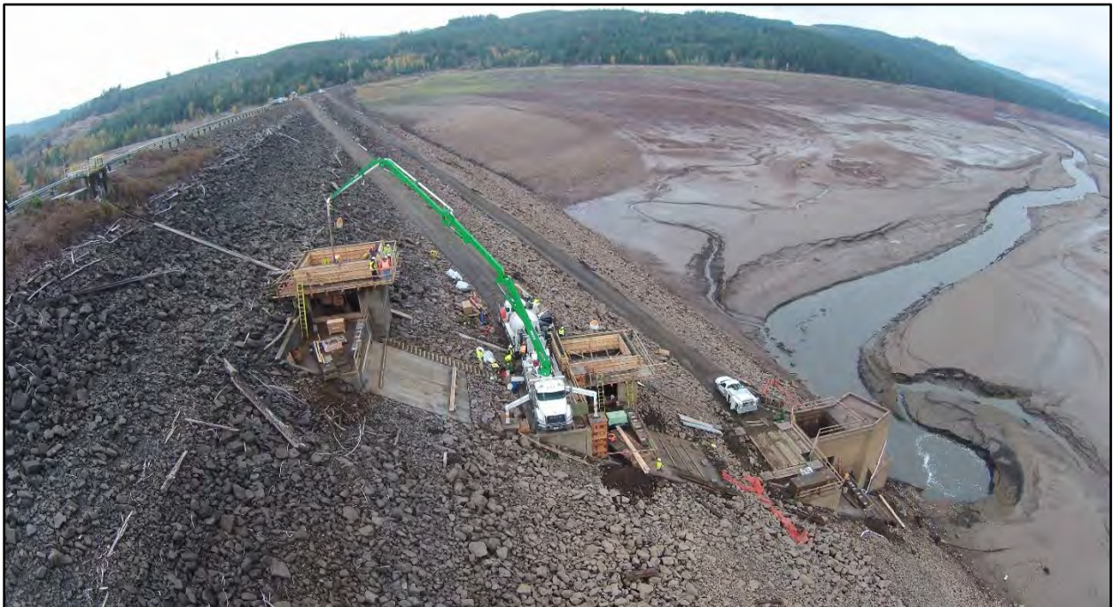
Figure 3.22-9. View of Fall Creek Dam and Reservoir during a deep reservoir drawdown to 10 ft above the ROs (USACE No Date-o)
