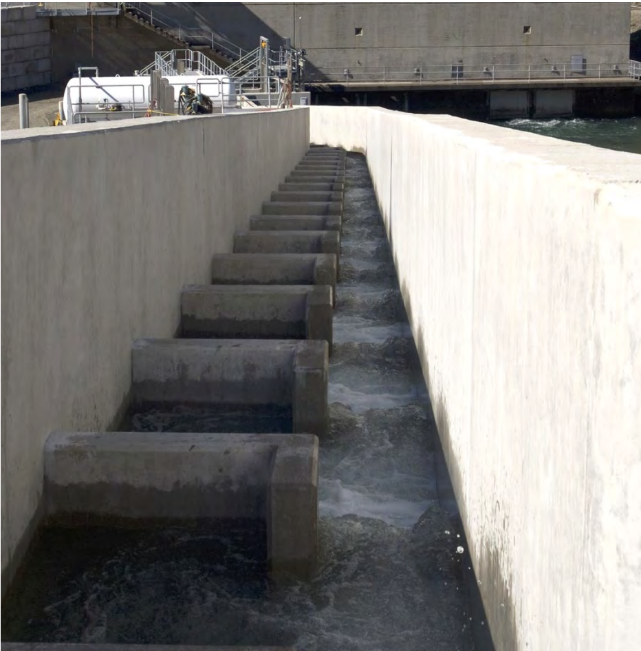
Figure 2.2-15. Fish Ladder at the Cougar Adult Fish Collection Facility
