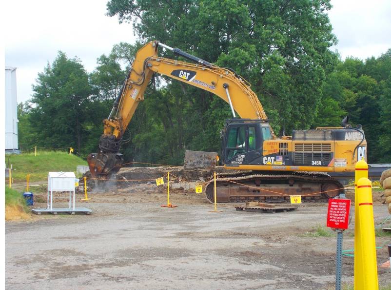
An excavator is used to remove soil, structure debris, and load them into waste containers to be shipped off-site for disposal.
