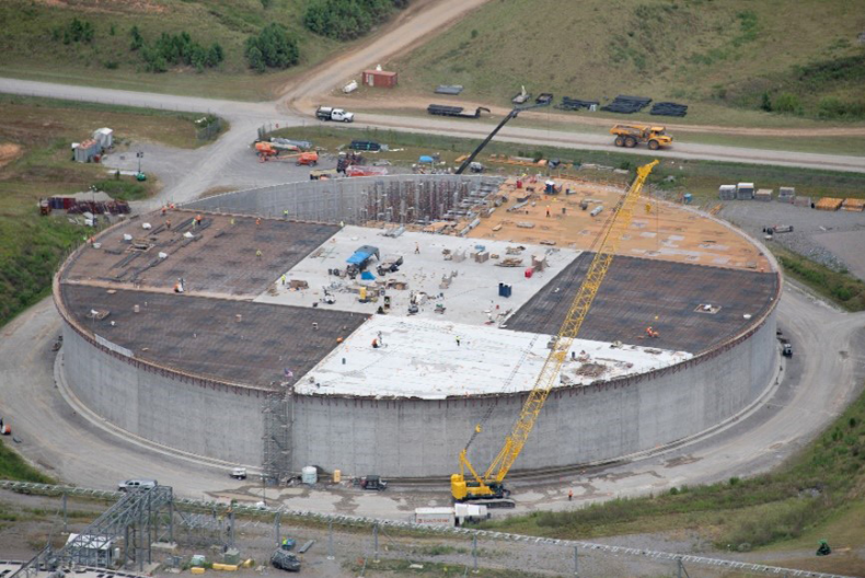
Workers in progress of completing all concrete placements on Saltstone Disposal Unit 9.
