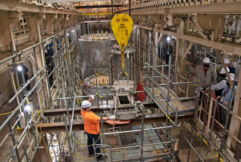
An electrolytic dissolver, used to dissolve stainless-steel clad fuel, was installed in H Canyon.
