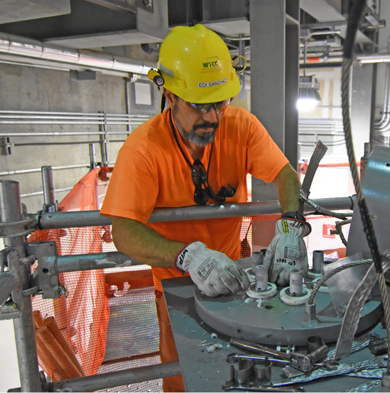
A Vit Plant electrician assembles temporary heaters that started up the first melter inside the plant's Low-Activity Waste Facility at the Hanford Site.
